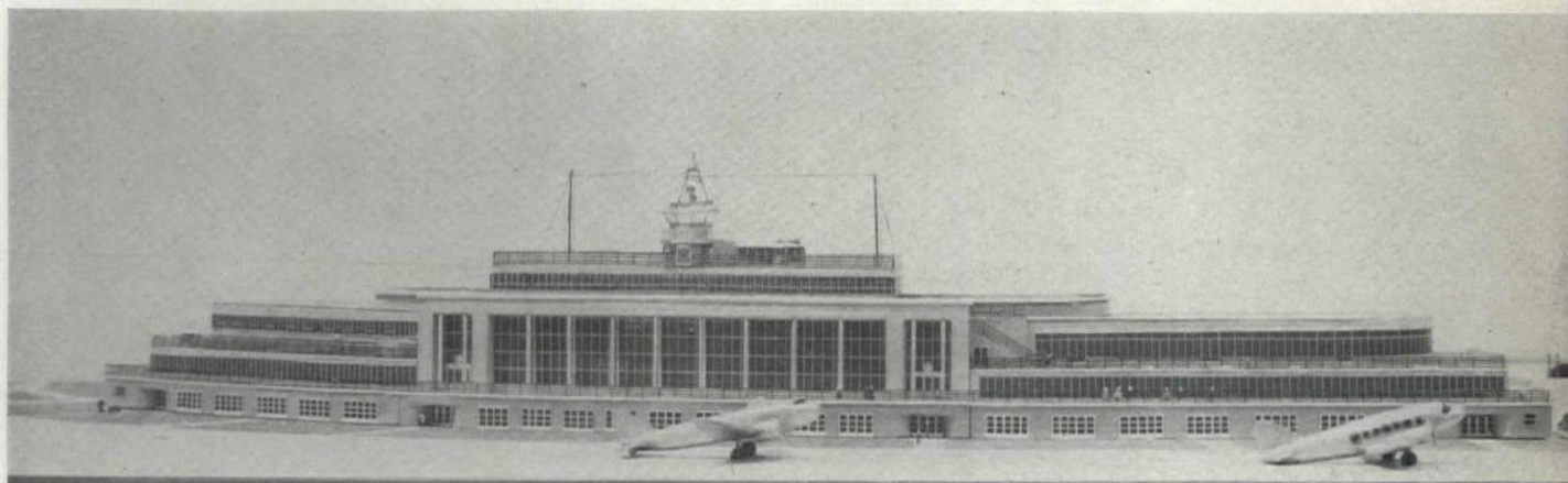
THE TERMINAL BUILDING AT WASHINGTON NATIONAL AIRPORT, AS IT WILL APPEAR FROM THE FIELD SIDE, SHOWN BY MEANS OF AN ACCURATE SCALE MODEL. ALMOST CONTINUOUS GLAZING IS SO ARRANGED AS TO INSURE UNOBSTRUCTED VIEWS OF THE FIELD FROM PRACTICALLY EVERY PART OF THE INTERIOR
