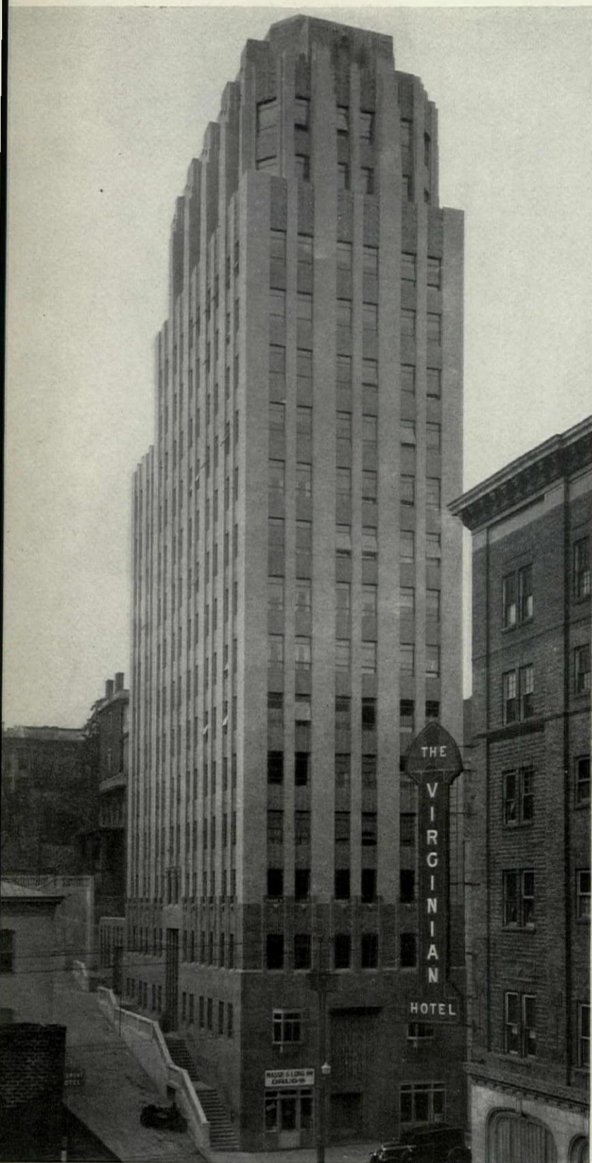
THE STRUCTURAL FRAME WAS ALL-WELDED WHEN THE ALLIED ARTS BUILDING IN LYNCHBURG, VIRGINIA (ABOVE) WAS BUILT. THE ARCHITECTS WERE JOHNSON & BRANNON, OF LYNCHBURG. THE WELDED FRAME PERMITS A CONSIDERABLE REDUCTION OF THE REQUIRED STEEL TONNAGE WHEN BUILDING A MULTIPLE-STORY STRUCTURE
