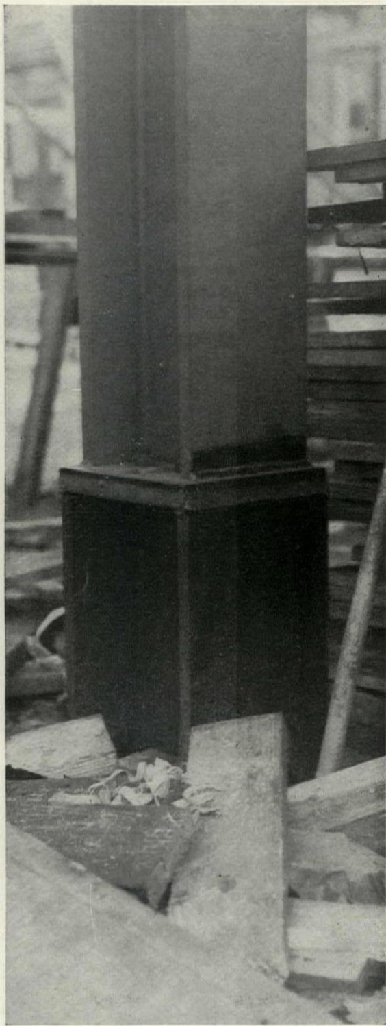
TYPICAL WELDED COLUMN CONNECTIONS
