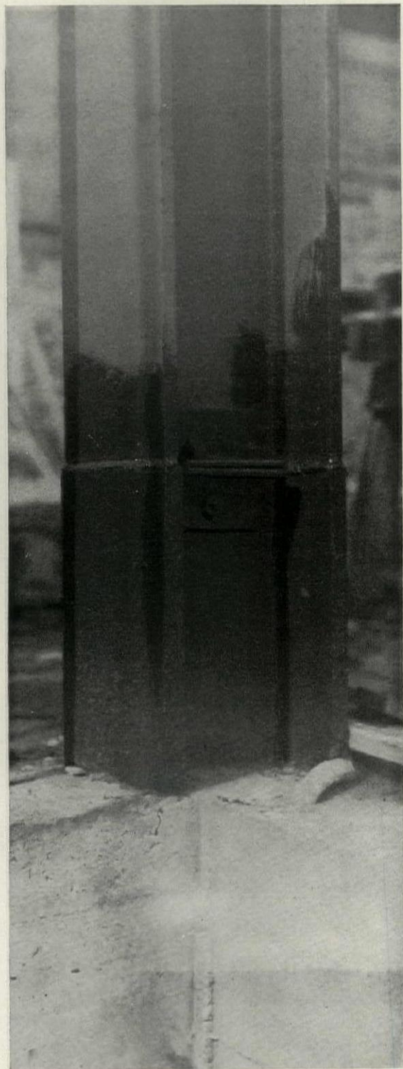
TYPICAL WELDED COLUMN CONNECTIONS
