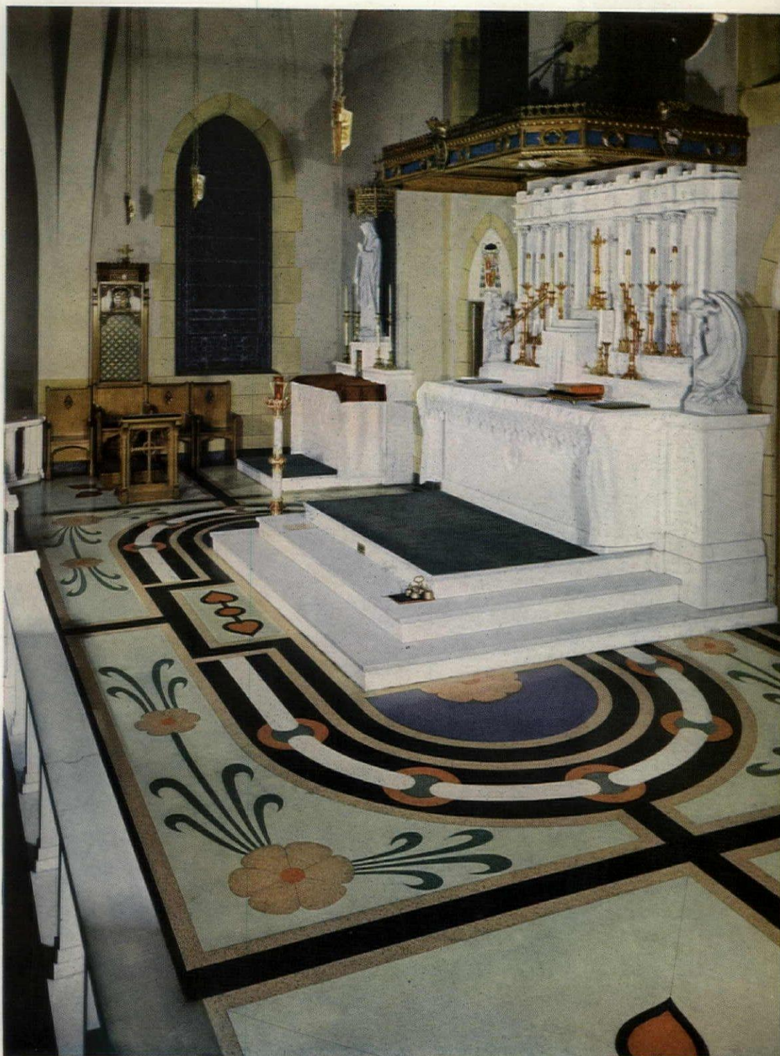
Beautiful floor in the Sacred Heart Cathedral, Raleigh, N. C. Marble aggregates used were: domestic white; Belgian Black with black pigment; Royal Green; Red Rosa with red pigment; and red fused enamel. Architect, F. Frimmer, St. Petersburg, Fla.; Terrazzo Contractor, Atlantic Marble and Tile Co., Inc., Charlotte, N. C.
