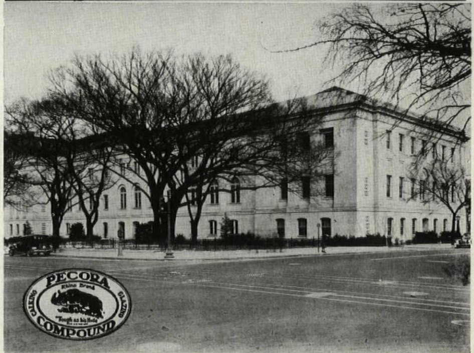
District of Columbia Police Court, Washington, D. C. Consolidated Engineering Co., Builders, Municipal Architect, Calked with Pecora Calking Compound by Chamberlin Metal Weather Strip Co., Washington, D. C.
