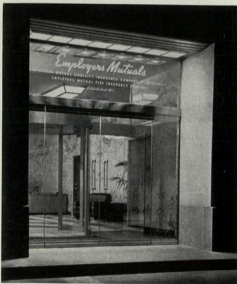
Three-story ornamental iron grilles, double-hung aluminum windows, Greenstone spandrels trimmed in extruded aluminum sections, and Herculite doors (detail below) are features of the Street Façade
