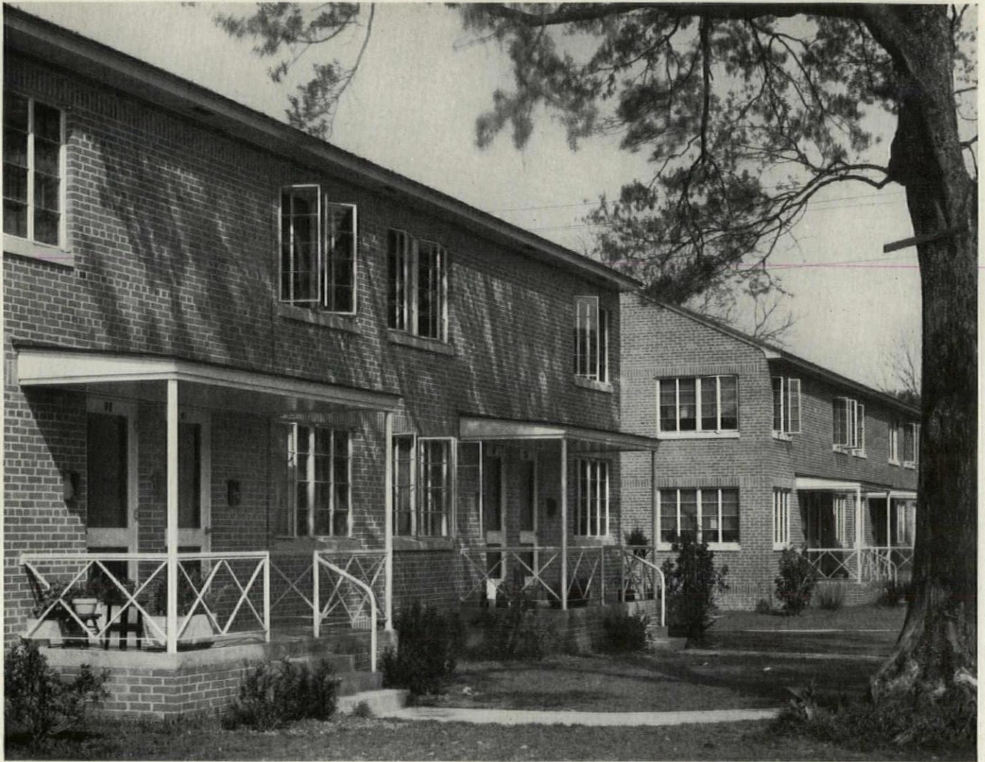
The "Oak Lawn Homes" units are constructed of brick on structural tile. Included in this project are four one-story buildings containing three-room apartments, and eight two-story buildings containing 4½- and 5½-room apartments, all grouped about the play area behind the Administration Building. (Richard W. Tebbs photos)
