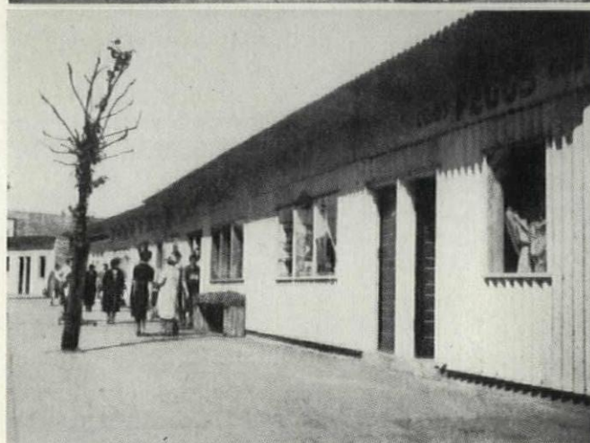
Temporary shops in Coventry are built of 2" x 4" wall studs covered on the outside with corrugated asbestos-cement sheets, inside with wallboard. Shops are designed back to back with roofs falling to a center-line box gutter. Remodeling by D. E. E. Gibson, City Architect. Photos from "The Builder," and "The Architect & Building News," London
