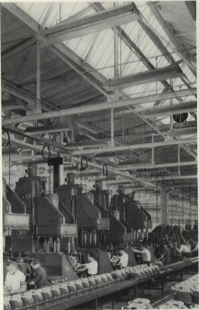
Section at 1 Section at 2 Non-glare glass was used in the factory monitors, which can be blacked-out with corrugated iron covers
