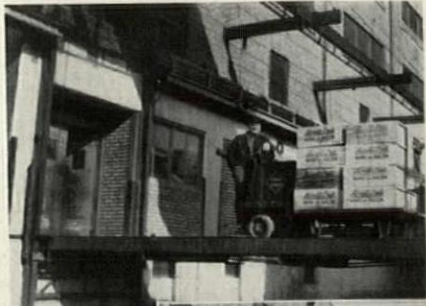
One of 5 Montgomery "Cross-Over" Bridges serving John Morrell & Co. Above: "Cross-Over" Bridge lowered. Right: "Cross-Over" Bridge raised for switching.
