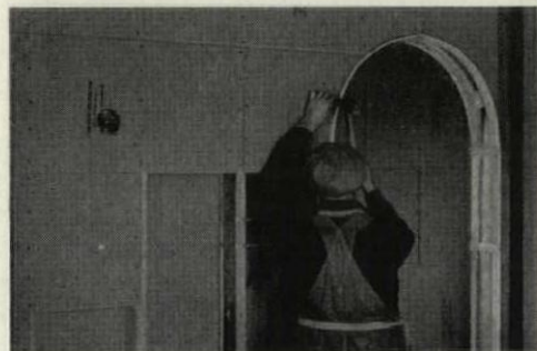
▲ LARGE BOARDS of Temlok Lath are quickly and easily nailed to joists and studding. They provide efficient, lasting insulation, and a strong, firm, and permanent base for plaster finish (exceeds U. S. Commercial Standards).
