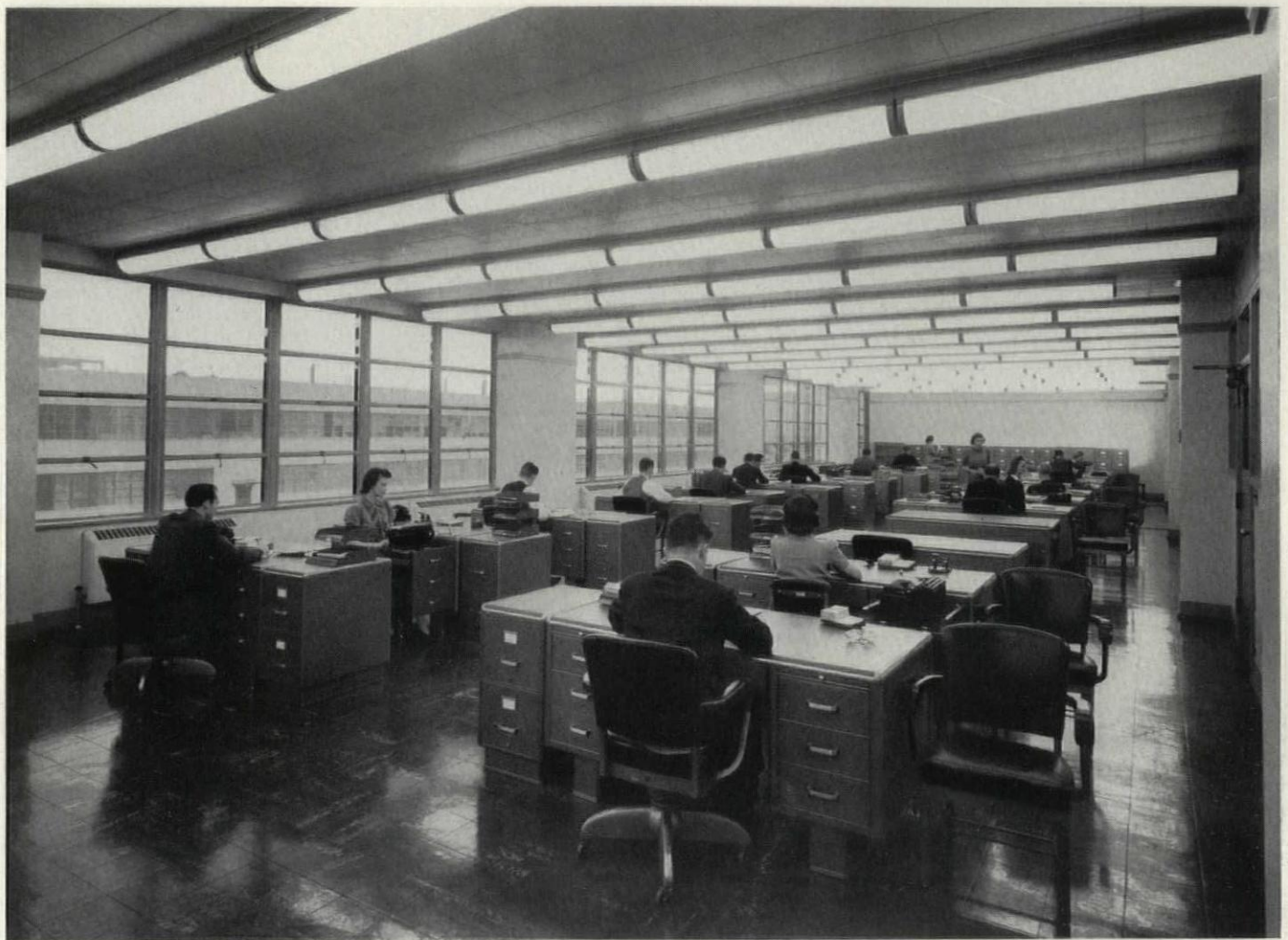
Lighting is also a prime consideration in the Clerical Departments, as this photograph shows. The ceilings and floors are sound-absorbent and all of this portion of the plant is air-conditioned. The plans (below) indicate efficiency of the administrative set-up, also on a "straight-line production" basis
