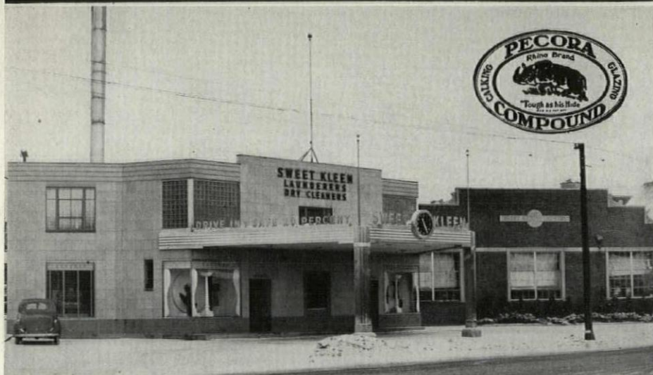
Sweet Kleen Laundry, Buffalo, N. Y. Hydro Const. Co., Buffalo, Genl. Contrs. Roswell E. Pfohl, Buffalo, Architect. Calked with Pecora Calking Compound by Niagara Metal Weather Strip Co., Buffalo, N. Y.
