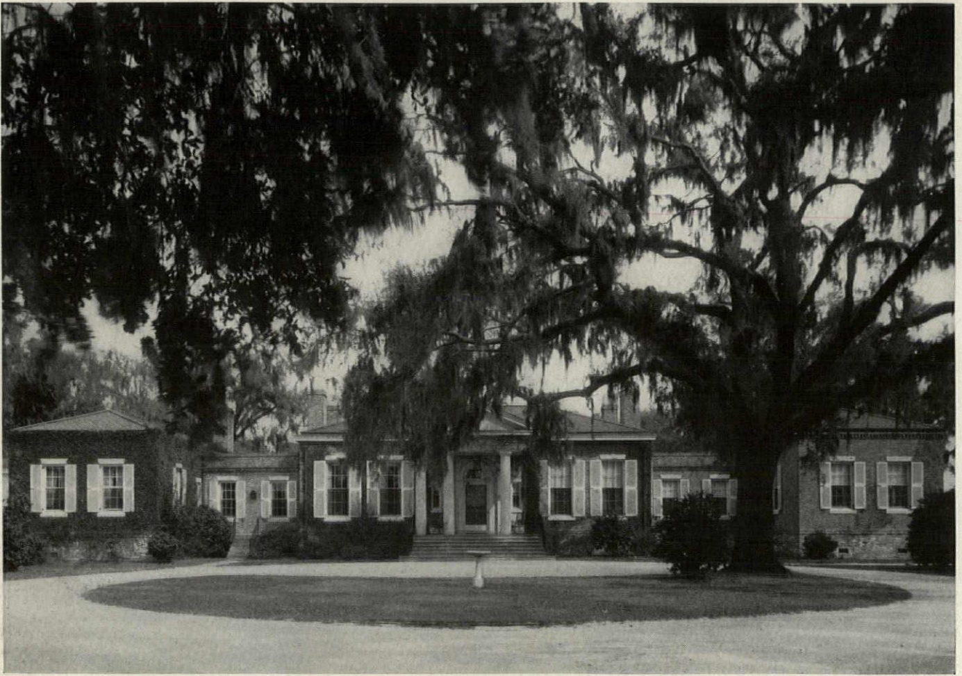
Situated approximately two miles from the public road, the building is approached through a grove of moss-hung live oaks of enormous size. The driveway ends in a circle at the entrance steps. (See Portico detail across-page.) Robert W. Tebbs photos
