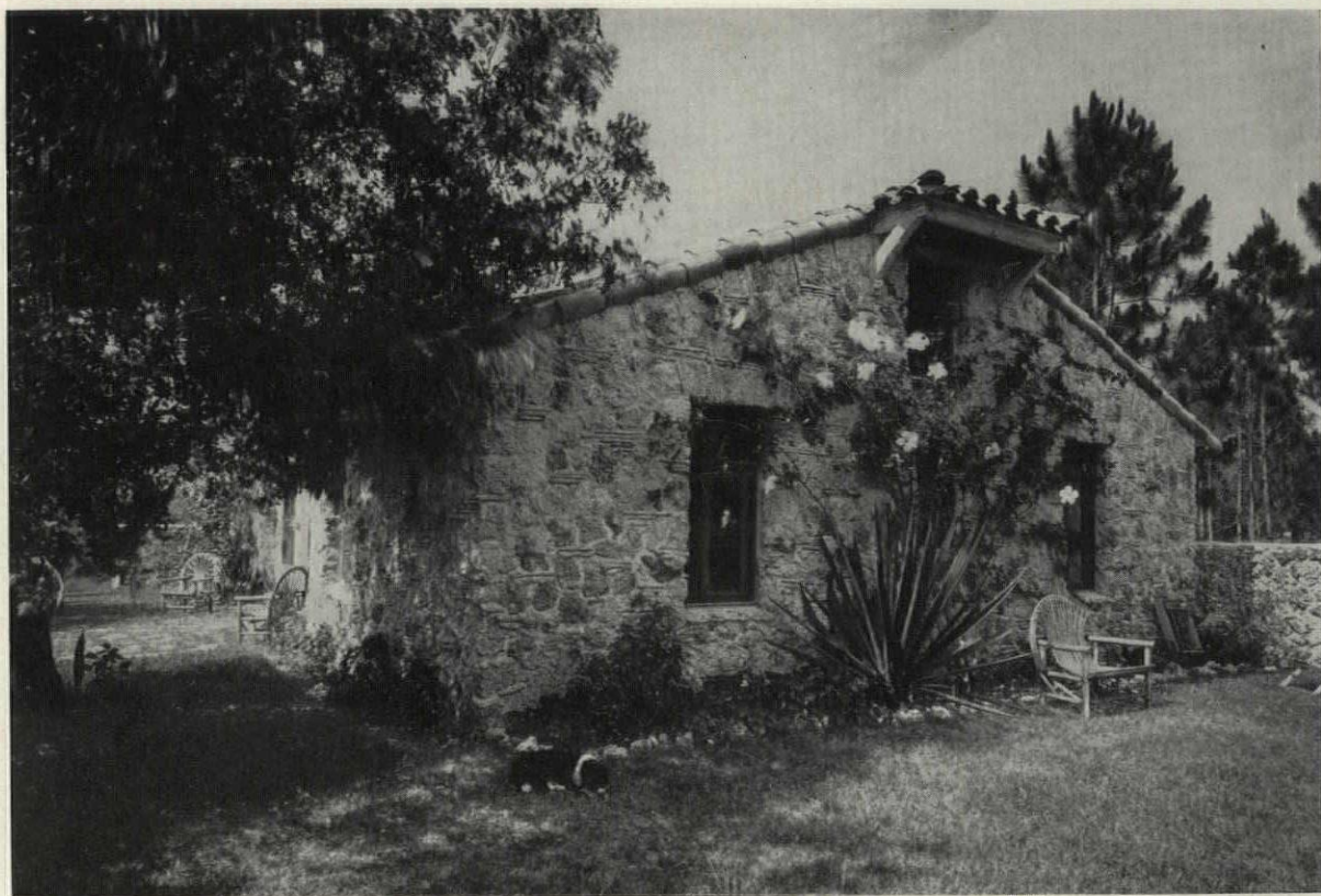
The walls are of coral rock, laid with random strips of red tile placed horizontally. Walls of the Patio, which is paved and screened, (below) are whitewashed coral rock. The roof is of Cuban tile
