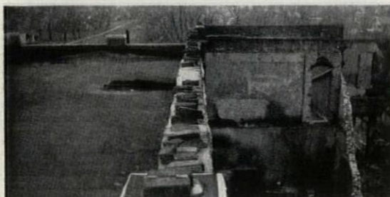
Although the low fire wall of the bank offered little protection, the flames were stopped by the J-M Asbestos Roof.
