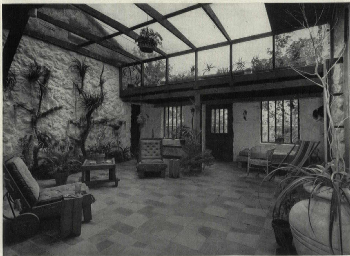
Screening is nailed to the exposed cypress frame. All the interior walls and ceilings are of cypress DESIGNED BY E. DEAN PARMELEE, ARCHITECT, OF MIAMI
