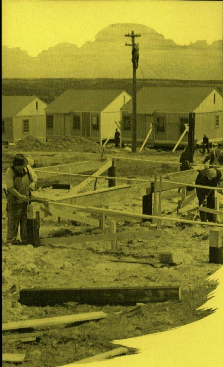
Halifax prefabricated houses are started on cedar post foundations.
