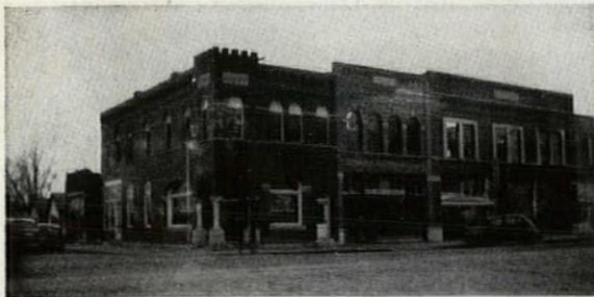
Starting in the building at the right, fire gutted the next two structures (see photo below), but a J-M Asbestos Roof saved the bank on the corner.
