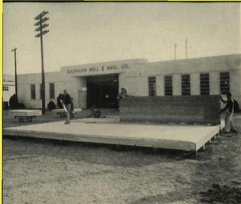
With sills and joists in place, floor panels are secured.
