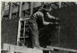
Attaching Wall Sheathing
