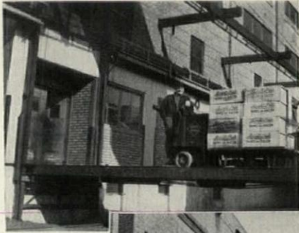
One of 5 Montgomery "Cross-Over" Bridges serving John Morrell & Co. Above—"Cross-Over" Bridge lowered. Right—"Cross-Over" Bridge raised for switching.
