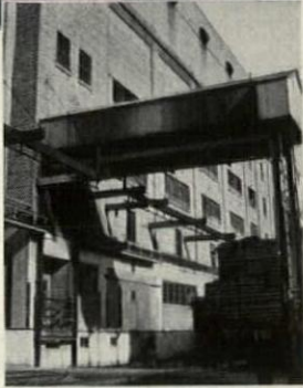
One of 5 Montgomery "Cross-Over" Bridges serving John Morrell & Co. Above—"Cross-Over" Bridge lowered. Right—"Cross-Over" Bridge raised for switching.
