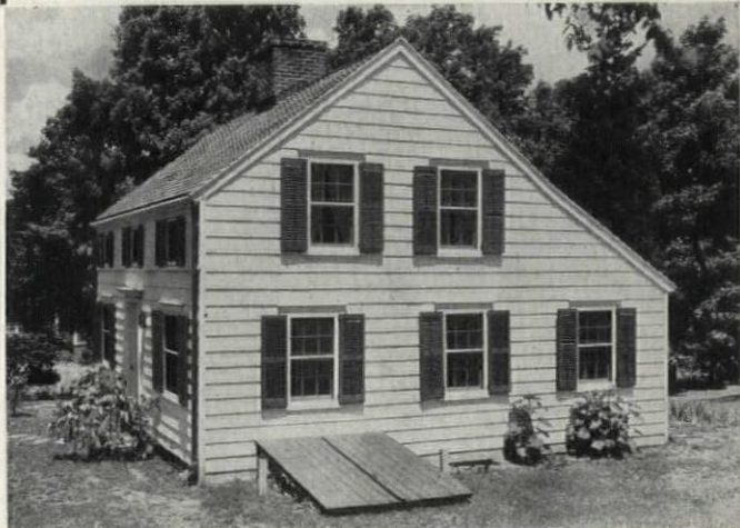
"Quilt" insulated house, Wilton, Conn. Architect: Evans Moore & Woodbridge
