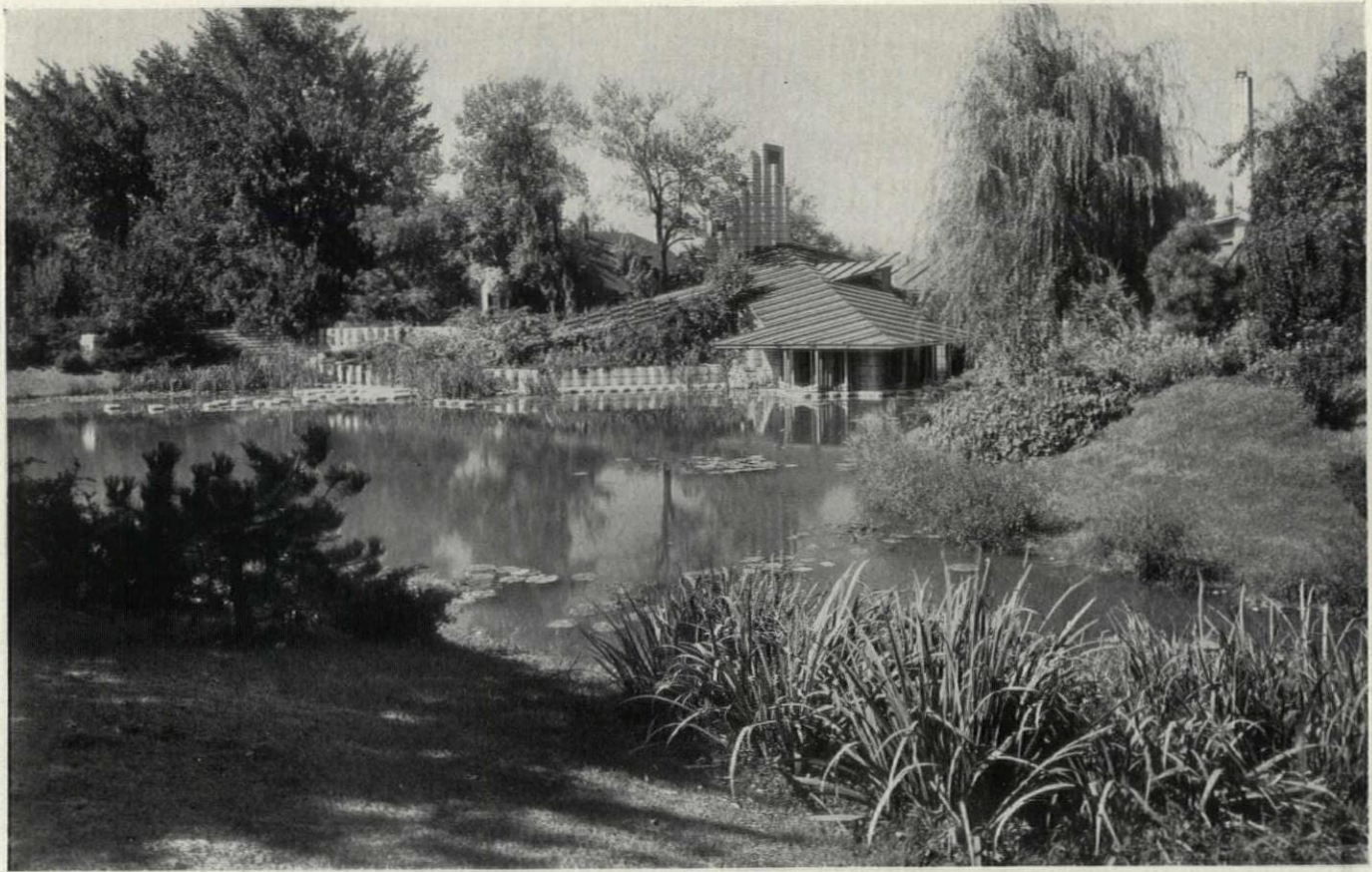
The rhythmically-lined slanting roof of the Dow Office (photograph above) gives evidence of the architect's skill in relating building with landscape. The integration of the exterior and interior, by using some of the exterior materials within, is reflected in the Consultation Room of the Office (lower photograph at right)—in the furniture, in the dramatic contrast of wood and cement block, in the lines of the cement block itself
