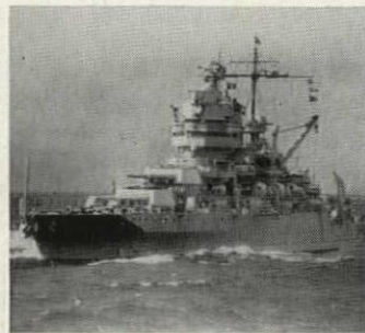
BATTLESHIPS are a maze of pipe and tubes. From stem to stern pipes provide strength and safety.
