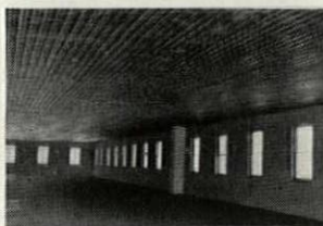
Diamond Rib Lath as Base for Plaster
