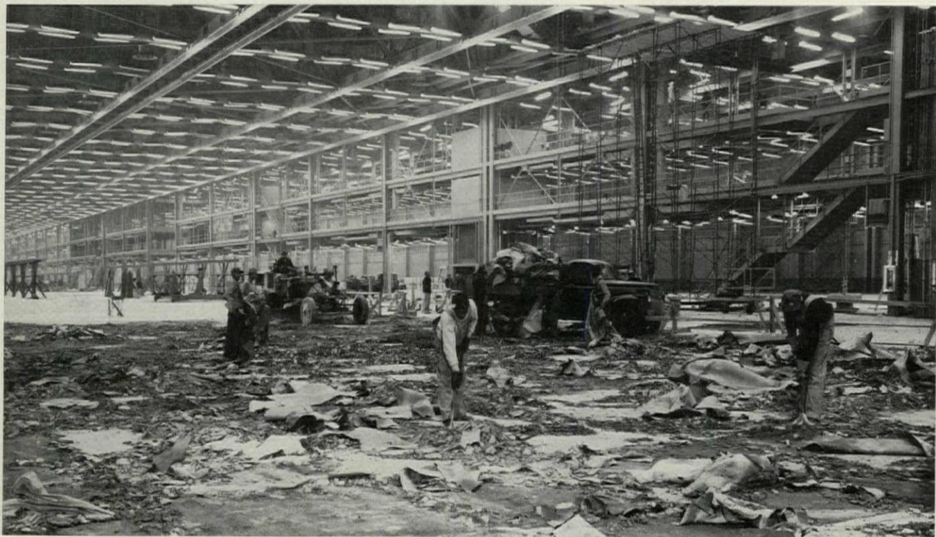
Above, light meter readings taken on adjoining areas of white and gray cement showed that the white floor reflected 44 per cent of the overhead light, the gray floor 27.4 percent. Below, workmen stripping the sand and paper protective layer from the white floor when construction of the plant was complete
