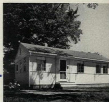
1941: FWA requests a "demountable" for defense workers. To meet nationally standardized requirements, a pitched roof, hinged to let down flat in transit, was added. Otherwise construction and erection were similar, sections were trucked from assembly line to foundations, rolled onto foundations on 4½-inch wheels mounted in the floor framing.
