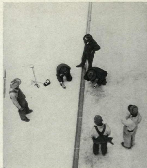
Above, light meter readings taken on adjoining areas of white and gray cement showed that the white floor reflected 44 per cent of the overhead light, the gray floor 27.4 percent. Below, workmen stripping the sand and paper protective layer from the white floor when construction of the plant was complete
