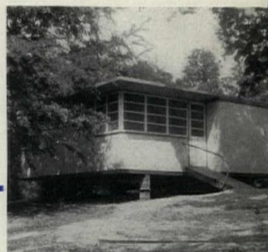
1940: The first sectional houses built for truck transport. Prefabricated in units 7½ feet wide, 22 feet long, 9½ feet high, each weighing about 3 tons, these can move over highways in most states on 2- or 4-wheeled trailers hauled by light trucks. Techniques developed on this project have been applied to all subsequent "demountable" houses built by TVA.
