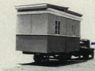
1941: FWA requests a "demountable" for defense workers. To meet nationally standardized requirements, a pitched roof, hinged to let down flat in transit, was added. Otherwise construction and erection were similar, sections were trucked from assembly line to foundations, rolled onto foundations on 4½-inch wheels mounted in the floor framing.
