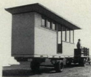
1940: The first sectional houses built for truck transport. Prefabricated in units 7½ feet wide, 22 feet long, 9½ feet high, each weighing about 3 tons, these can move over highways in most states on 2- or 4-wheeled trailers hauled by light trucks. Techniques developed on this project have been applied to all subsequent "demountable" houses built by TVA.
