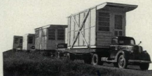
1941: Same construction-for-portability principles for TVA's own housing, but more economical plans. As in all TVA portable houses, electric, heating, plumbing equipment is pre-installed; almost no loose building material is needed for assembly. Six men can unload and assemble a two-section house in 2 hours. Original cost per house, $1900. Trucking costs: 30c per mile per section; total moving cost for 34 miles, $280 per house including all site work except extending utilities.
