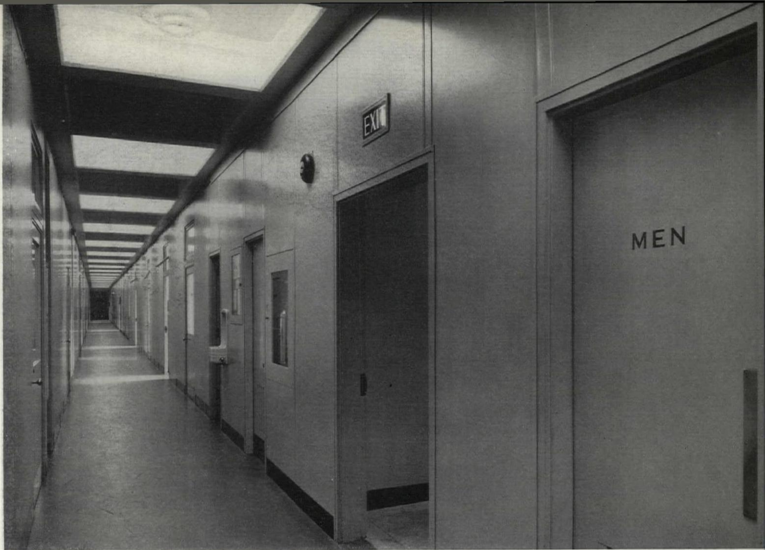
A typical laboratory corridor which shows clearly the standard metal wall units and also the method of lighting. Corridors in chemical laboratory are equipped with emergency shower heads for extinguishing burning clothing. These occur at 48-foot intervals and operate by pull-chains within easy reach
