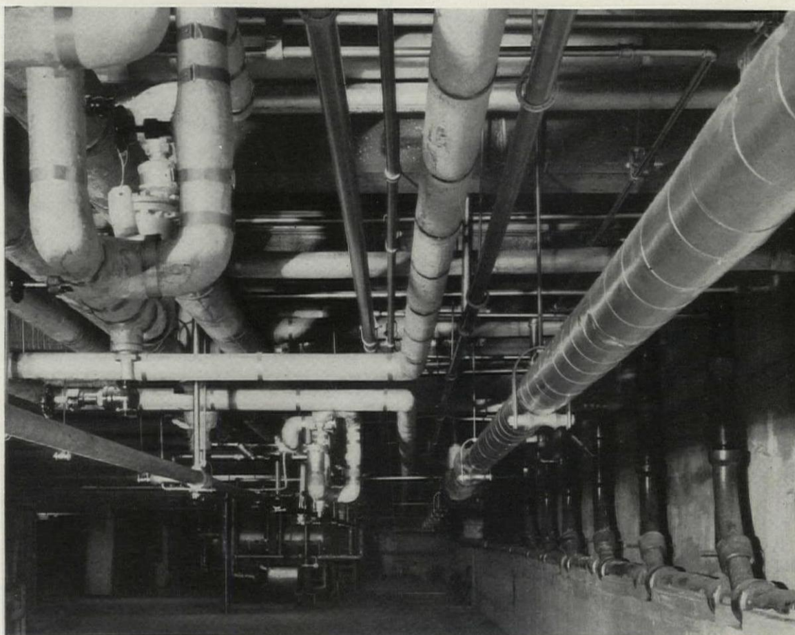
Actual engineering study combined with the experience gained in the test house made possible the installation of basement loop services, properly spaced and fitted. Note the drains on 6-foot intervals for each module plan unit of the superstructure. Section above, (right) shows typical arrangement of loop service piping in the basement as related to the typical service distribution on the first floor. The local horizontal distribution for typical floors is below the window, between the radiator enclosure and the exterior of the metal wainscot
