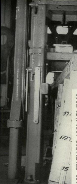
FIG. 6. Plywood girder failed by buckling laterally under a load of 110,580 lb.—many times the design loading
