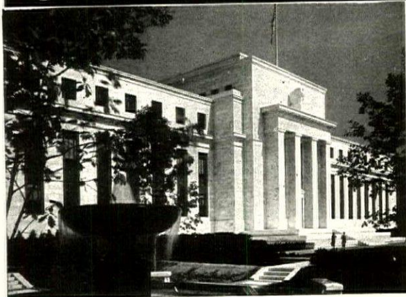
The Federal Reserve Board Building in Washington, D. C., is one of an impressive list of Federal buildings throughout the country calked with Pecora.
