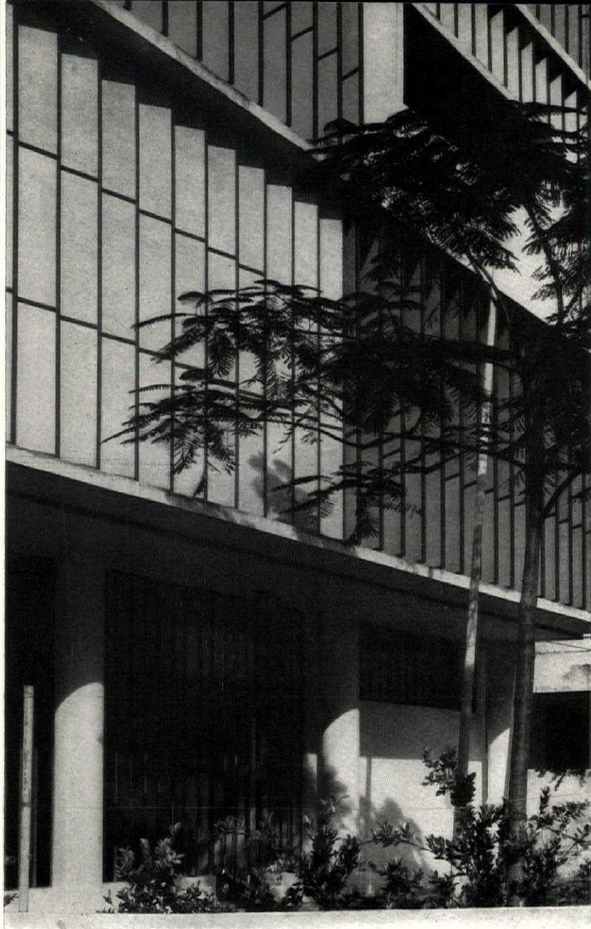
Obra do Berço (Nursery) at left above and below, Oscar Niemeyer, Architect; Boat Passenger Station, right above, Corrêa Lima, Architect. In both buildings the louvers are movable, and are supported between horizontal or vertical concrete fins. Corrêa Lima's louvers in the Station are similar to those on the Ministry of Education and Health. The Obra do Berço louvers are approximately 6 feet high by 1 foot wide, crank-operated.
