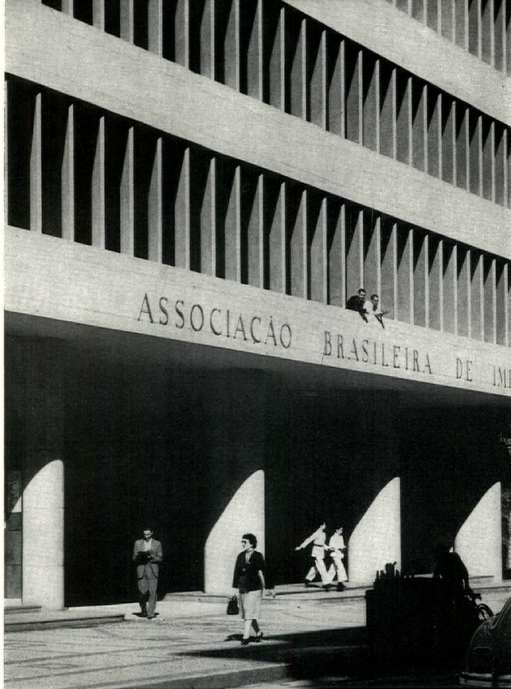
The ABI (Brazilian Press Association) Building in Rio de Janeiro was designed by Marcelo and Milton Roberto, Architects. Louvers here are of concrete, fixed. At street level the lobby is completely open. Photos by G. E. Kidder-Smith, AIA. Details, indicating how the louver principle—called in Portuguese quebra sol , but more generally designated by the French term, brise-soleil —operates, are shown on pages 62 and 63.
