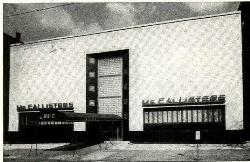
Insets in panels supply an interesting note; McCallisters, Caterers, Philadelphia, Pa.; Black Serpentine bulkheads and panels; Armand Carroll, Architect.
