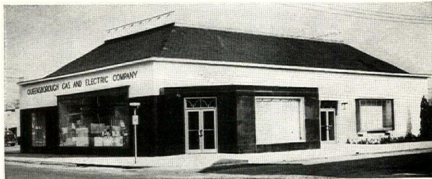
Distinctive Valley Stream, N. Y., Branch Bldg., Queensboro Gas & Electric Co.; Voorhees, Walker, Foley & Smith, Architects; Black Serpentine facing and bulkheads.
