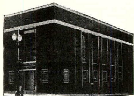
Sheer facades of Black Serpentine; Central Bank of Grand Rapids, Mich.; Knecht, McCarthy & Theband, Inc., Architects.
