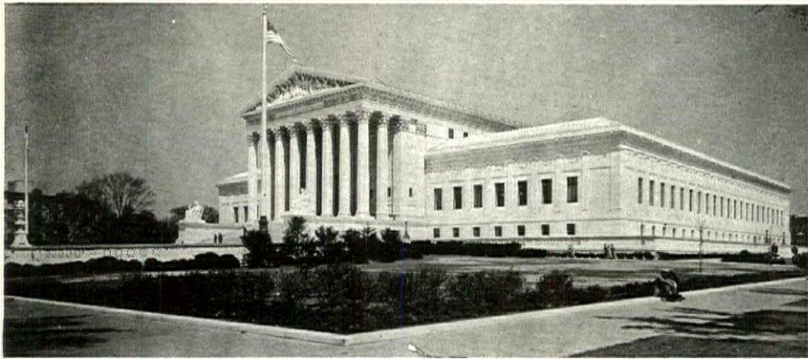
The Supreme Court Building in Washington, D. C., is one of an impressive list of Federal Buildings throughout the country calked with Pecora.
