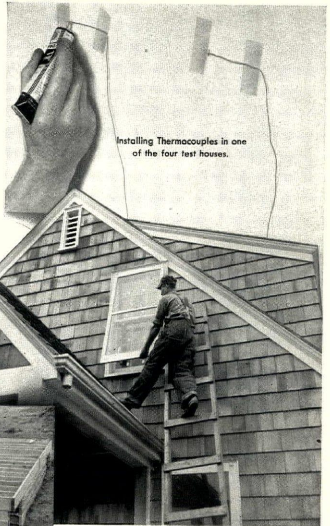
Installing storm windows on a test house.
