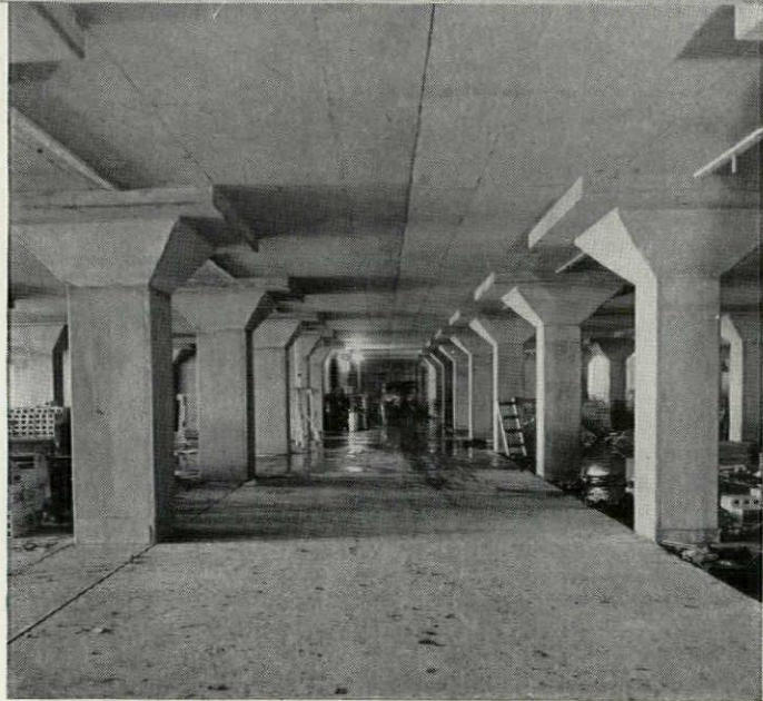
All-concrete Administration Building of arsenal in middle west. Designed by U. S. Engineer Office. Priester Const. Co., Davenport, Iowa, contractor.
