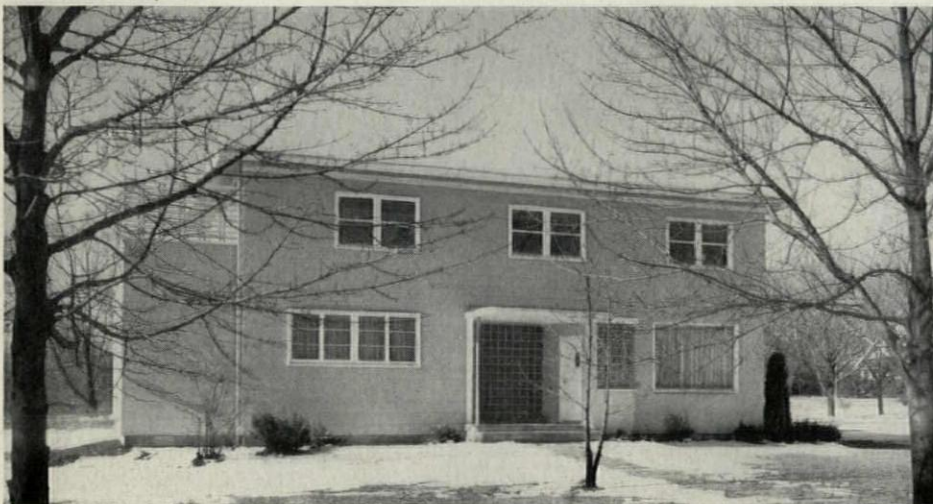
Exterior is faced with Redwood in a neutral gray color, with narrow white trim and a turquoise blue cornice soffit. Marquis soffit is stucco, terra cotta colored.
