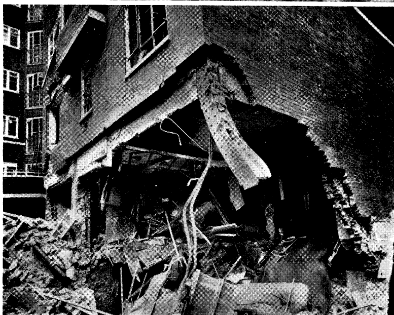
1. Steel-framed structures show the ability to withstand severe punishment from bombing without disintegrating as is the case with plain masonry structures.
