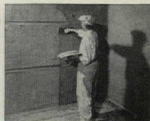
Then brown coat plaster is applied—followed by finish coat.
