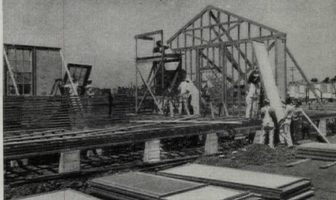
MODULOK CEMESTO WALL UNITS go easily into construction of a unit of the Naval Hospital at Corona, California. This is just one of hundreds of projects where Cemesto panels have been used.
