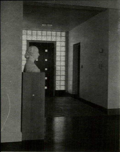
Main stair and floor of entrance hall are green slate, with natural cleft surface
