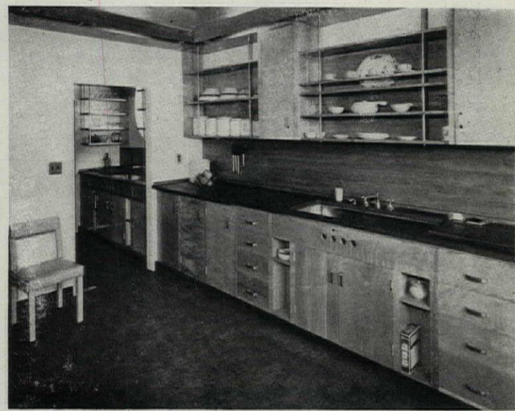
Kitchen and pantry cabinets and shelves are birch; treated with a solution of cellulose; work counters of teak are oiled
