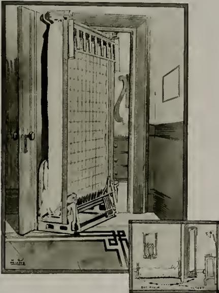
Swinging Bed Into Room. Showing Wall Section
