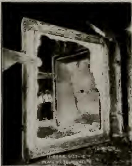
this construction might prevent the spread of a conflagration through a residential district. On the outer side of the studding, which would correspond to the inner
