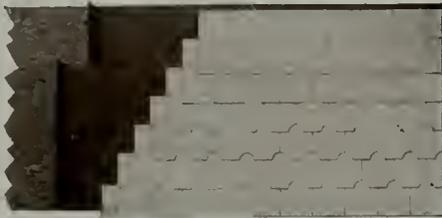
Nos. 72, 77 and 82 (priced on page 58 of the Asbestos "Century" Shingle Catalog), employed as a band course to break the straight and even lines when laid according to the "American" method. This style or shaped shingle is frequently used for siding, especially in the gables, etc.
