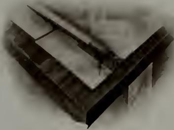
FIG. H.—STANDING-SEAM TIN ROOFING
