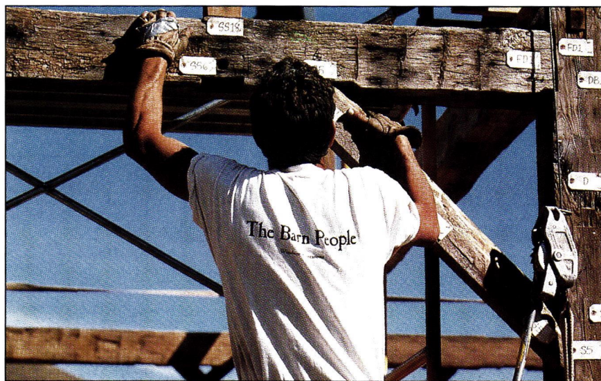
Detail of a 30-x-60-ft. bay barn, braced and tagged and ready for craning down.
