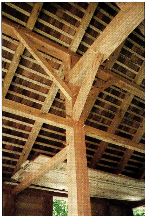
Adapting the Dutch anchor-beam framing method, ARCHITECTURAL TIMBERWORKS created this barn for an interpretive history site in Bergen County, New Jersey. Write in No. 592
