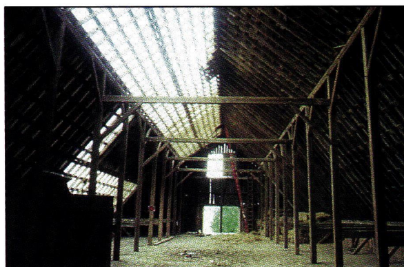
DEAN FITZGERALD HEAVY TIMBER CONSTRUCTION re-stored this barn roof with 2,000 board feet of custom-milled yellow poplar. They also replaced some heavy timbers and rafters. Write in No. 2300
