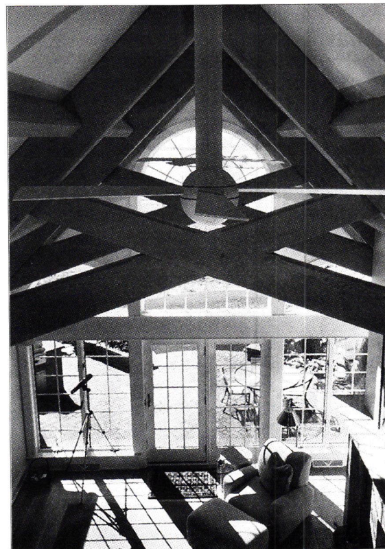
The roofing truss in this LANCASTER COUNTY TIMBER FRAMES home was made from recycled Douglas fir.
