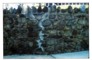
Fig. 2. A detail of Fig. 1 shows extensive repair work was needed. In fact, unless weep-holes are provided, this wall will come down in a few years.
