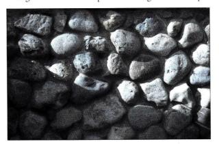
Fig. 3. An example of river-stone work showing some pleasing harmonies between individual stones, yet the wall remains static and lacks flow.
