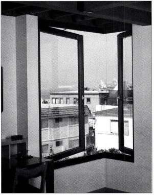
This European open-out casement, offered by ZELUCK, features a concealed locking system integrated with a special guide stay. Write in No. 6920
