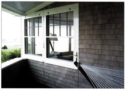
windows used an array of different systems, from ropes and pulleys to tapes and balances. Specs called for exterior storm windows and screens and, to eliminate the need for puttying, wood-stopped single glazing.
