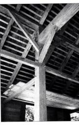
The Dutch anchor-beam barn style was adapted by ARCHITECTURAL TIMBERWORKS for this newly built display barn. Write in No. 592
