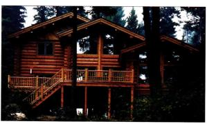
This home from PRECISION CRAFT LOG STRUCTURES was built in a Swedish cope style featuring beaver-tooth corners punctuated by interlocking saddle-notch corners.
