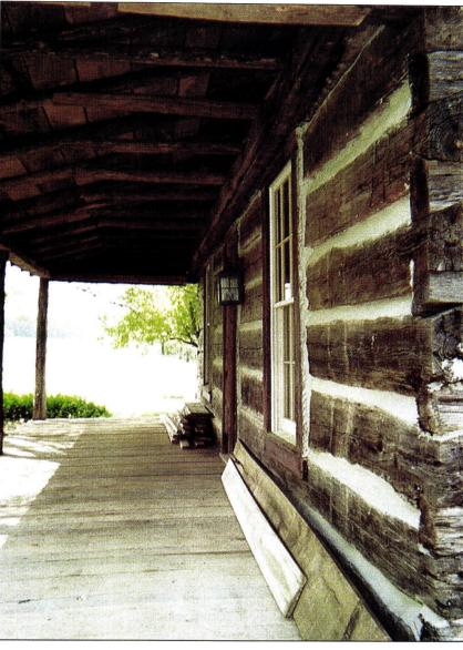
Above: This photograph shows up close detail work on a log cabin restored by Kerry S. Hix. This cabin originally was meticulously taken apart and reassembled. Part of Hix's expertise lies in the ability to reconstruct the hand-hewn elements without defacing the integrity of old timbers or losing the patinaed quality. (Photo courtesy of Kerry S. Hix Antique Log Cabins)
