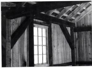
FITZGERALD HEAVY TIMBER CONSTRUCTION milled the timber for this frame using an antique Frick sawmill. Write in No. 2300
