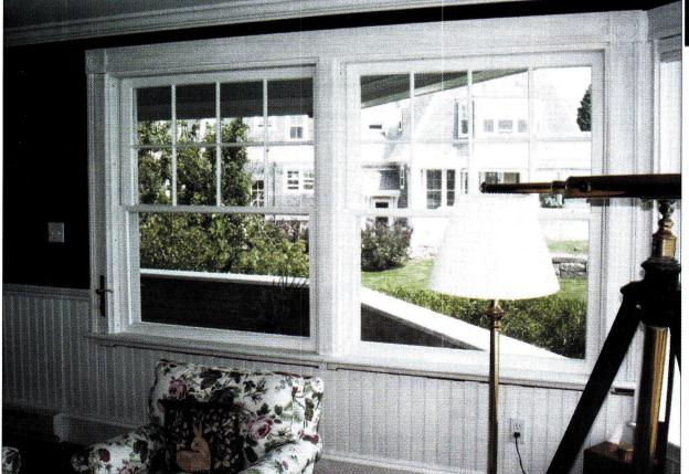
INTERIOR VIEWS Top left: When is this panel a door? When it's ajar. Basically complete — except for the interior molding beneath the glass — the panel swings open to the porch. Above: When the panel is closed, the hinges are invisible and the sills of the adjacent windows meet, creating a seamless appearance. Only the brass handle, at left, suggests the existence of a door.
