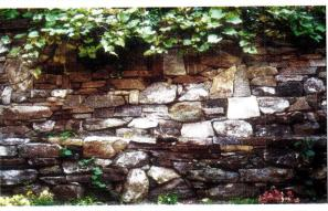
Fig. 14 (top). A heavy coating of enamel paint prevented drainage and caused this wall to collapse. Figs. 15 (middle) & 16 (above) illustrate the wall rebuilt without mortar, using various fieldstone. Notice the tight joints, the flowing lines within even courses, and the way in which each stone stands out.
