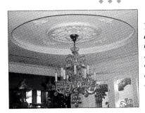
The dome effect in this ceiling was produced by using MANOR STYLE flex molding on the perimeter of a circular recess and adding a medallion.
