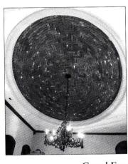
GRAND ENTRIES' striking elliptical brick dome has a minor axis of 12 ft., a major axis of 18 ft., and rises 32 in. at the center.
