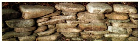
Fig. 9. Notice the long vertical joints, which weaken this poorly laid-up dry wall of river flats.
