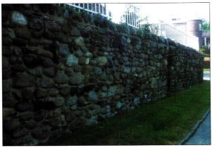
Fig. 1. This tall river-stone wall is built with inadequate drainage and little appreciation of the individual qualities of the stone.
