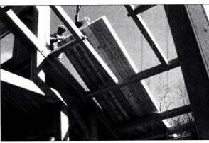
Woodclad structural insulated panels from WINTER PANEL can span up to 8 ft. in roof applications. Write in No. 672
