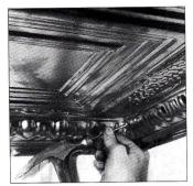
After a ceiling from AA-ABBINGDON has been nailed in place, caulk is used to hide the seams where the sections of metal meet. Write in No. 8920
