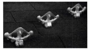
Primarily for installation on slate roofs, Gothic snowguards from G.T. Products are made of hot-dipped galvanized cast iron.
