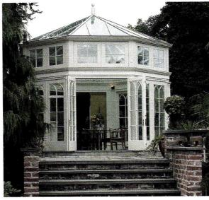
This glass house built by Tanglewood Conservatories features interior woodwork and maintenance-free aluminum cladding.
