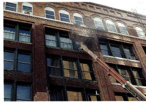
ArmaKleen manufactures Armex blast media, a baking sodabased abrasive for gently cleaning brick and other substrates.
