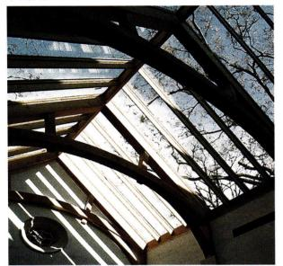
With this glass-roof system from Glass House, LLC, the molded timber-frame gable roof provides a light, airy transition to garden areas.
