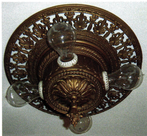
Al-Bar Wilmette Platers cleaned and re-wired this flush-mount original fixture for a building in Chicago.
