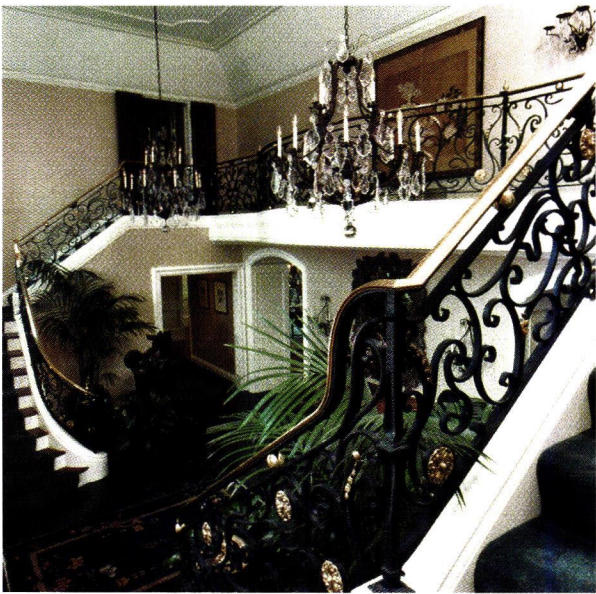
These forged-iron stairs and balcony railing — designed, fabricated and installed by Wiemann Ironworks for a residence in Wichita, KS — feature a polished-bronze cap rail, rosettes and decorative elements.
