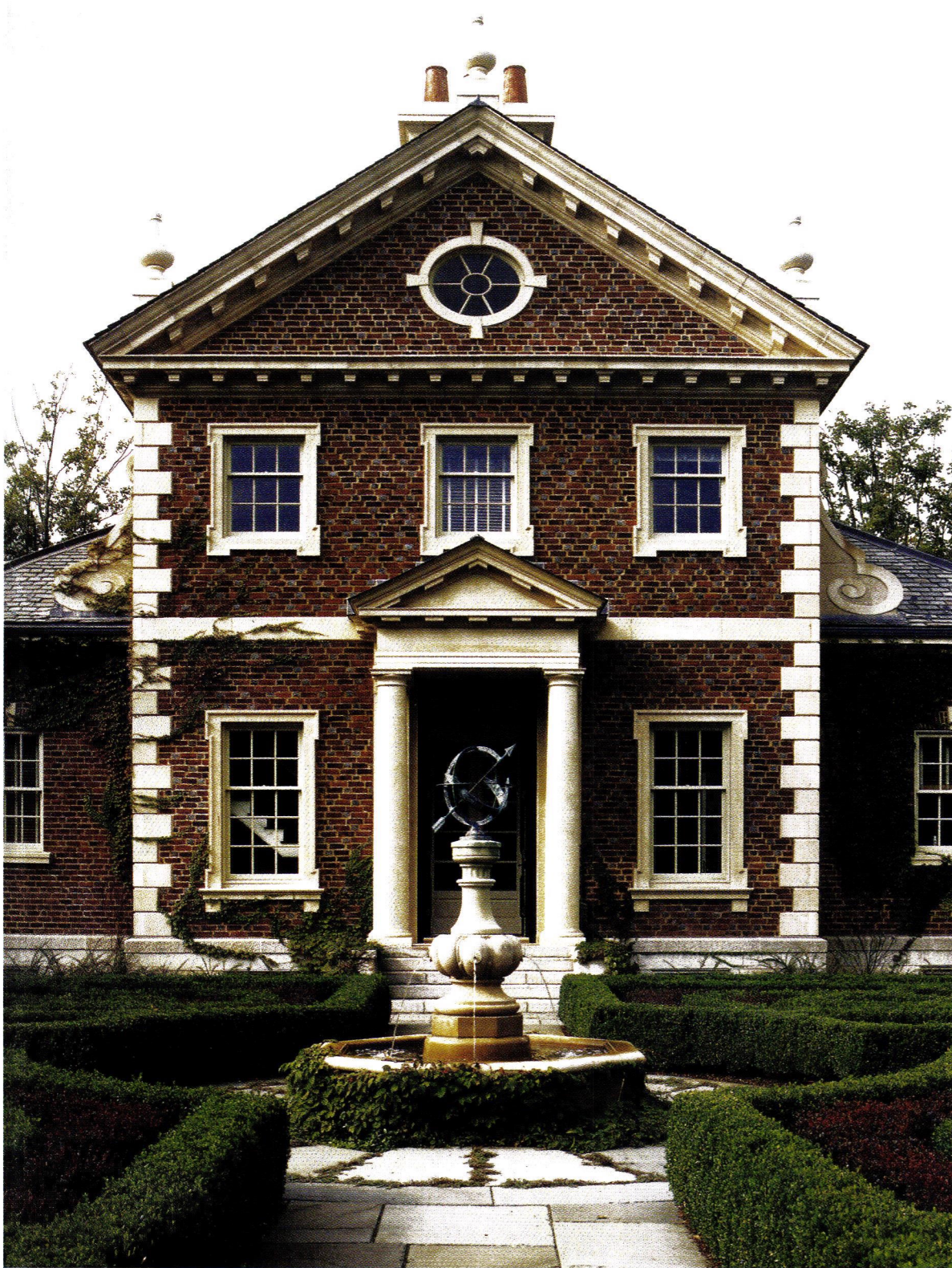
At a Palladian estate in Connecticut, multi-colored Virginia bricks mingle with blue-glazed headers and cast-stone ornament.
