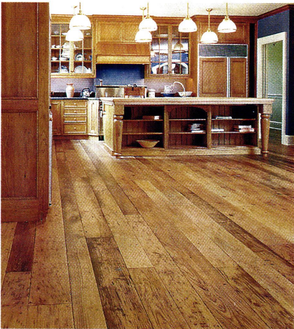
This random-width plank chestnut flooring was supplied by Chestnut Specialists and finished with oil and wax.
