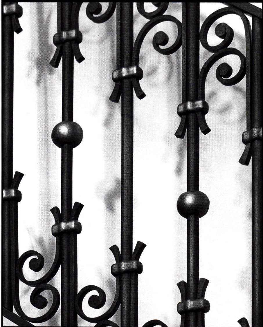
Forged iron stair railing with patinated finish and custom bronze collars and bands.
