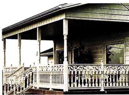
Newel posts and balusters from Vintage Woodworks are turned from clear, solid, kiln-dried western hemlock.
