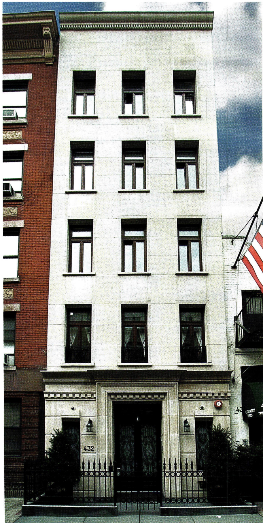
Kratchman added two stories and pinned French limestone to the brickwork. Two-inch reveals between limestone blocks give the base a sense of heft and depth. All photos: courtesy of Steven Kratchman Architect, P.C.
