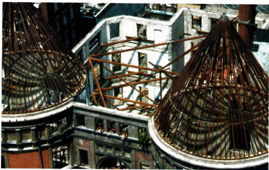
Above: Very little of the interior could be salvaged. Gutting the building involved bracing the walls with structural steel. Photo: RKT&B
