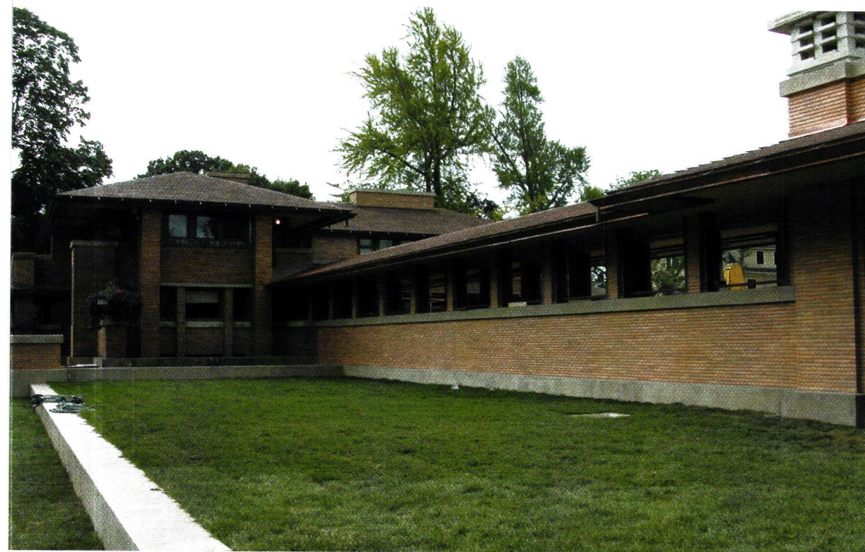
Roman bricks on a newly recreated pergola (right) match the existing cladding (left). Photo: courtesy of the Martin House Restoration Corporation
