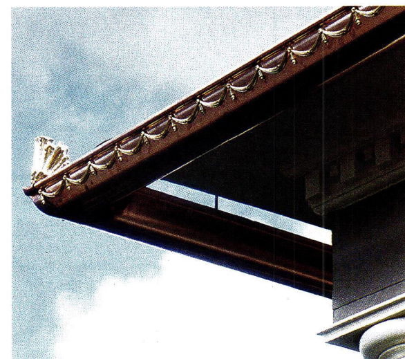
Classic Gutter Systems fashioned this elaborate half-round copper gutter with gold-patinated solid-brass trim and a rain deflector.
