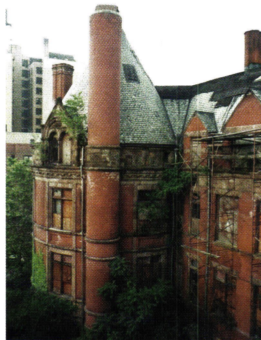
Between 1974 and 2001, the building was left vacant and fell into great disrepair. Much of the roofing slate was damaged or missing, the roof was caving in, the stonework was displaced or eroded, the windows were broken and vegetation had gained a foothold in the masonry, rotting the top five feet of the façade. Photo: RKT&B
