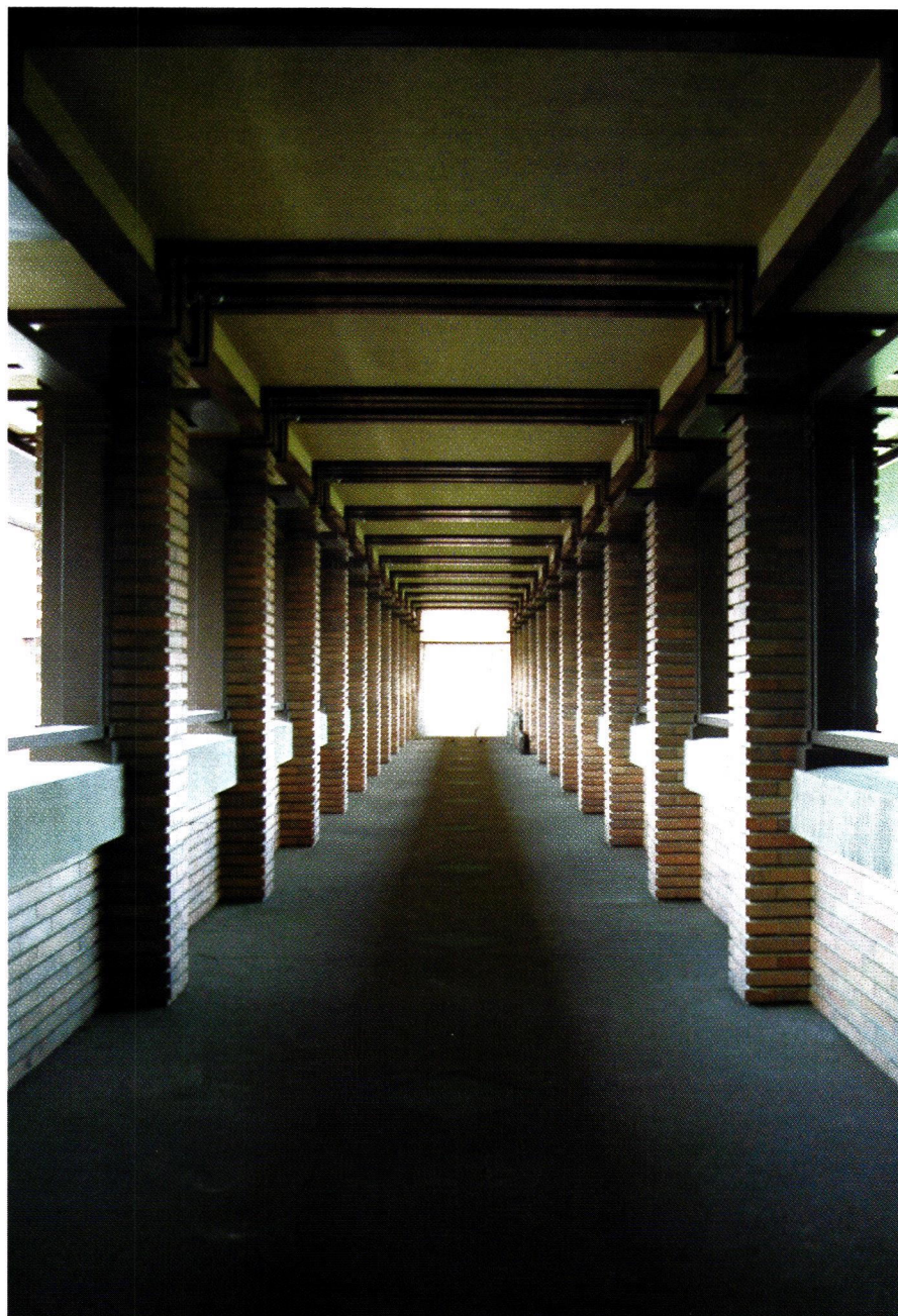
Oak beams and brick piers march rhythmically down the pergola. Photo: courtesy of the Martin House Restoration Corporation
