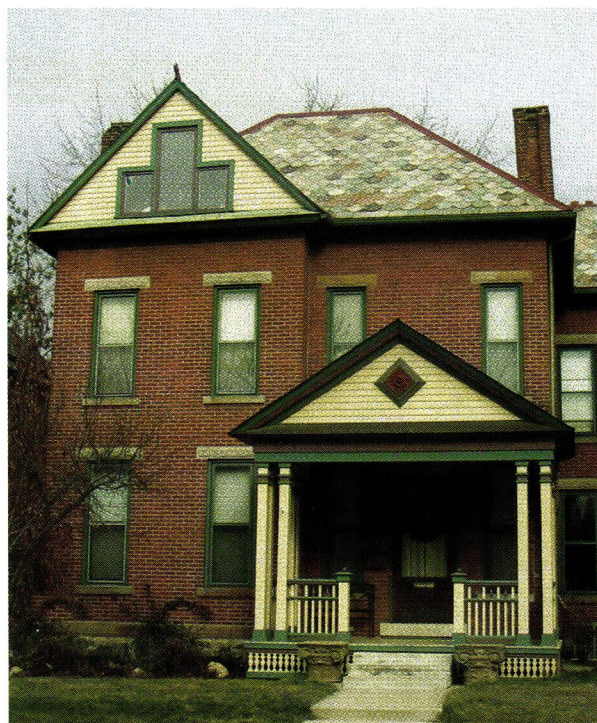
The Durable Slate Co. installed this slate roof using reclaimed Vermont semi-weathered gray-green and purple slates.
