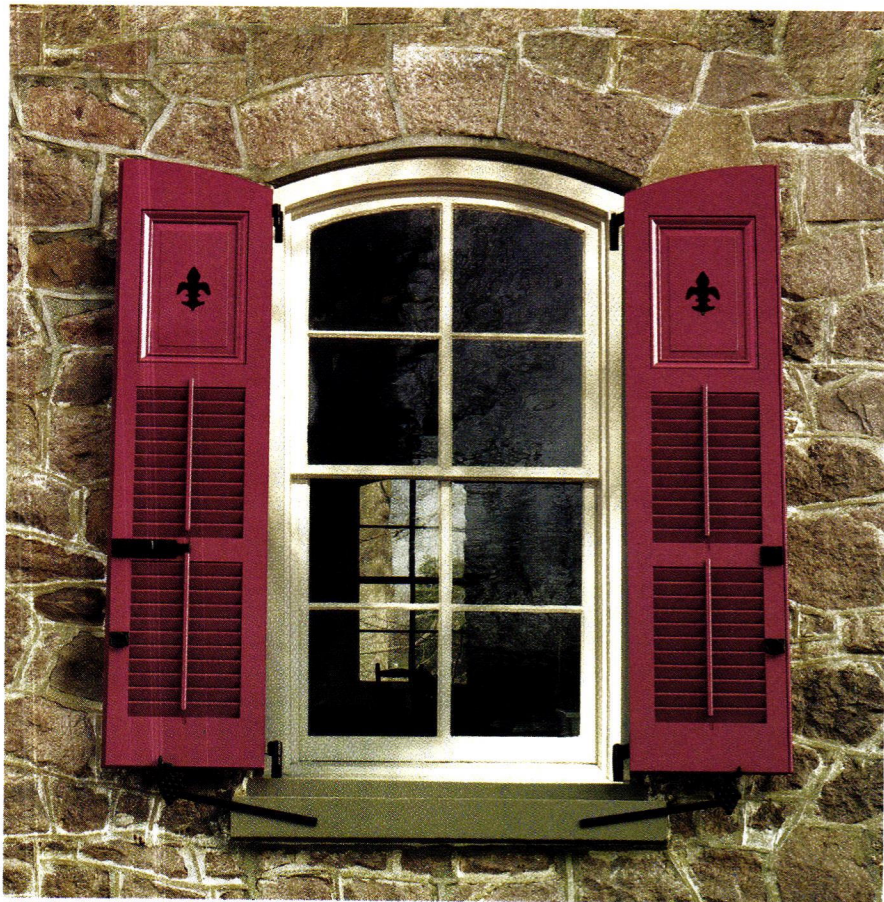
These western red cedar combination shutters from Timberlane feature a louver bottom and a raised-panel top with a fleur-de-lis cutout. Photo: courtesy of Timberlane, Inc.
