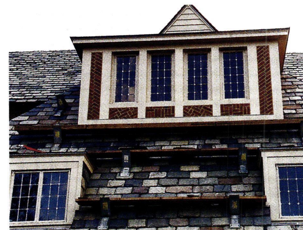
These 75-year-old steel casement windows were salvaged and then incorporated into this structure by Seekircher Steel Window Repair.
