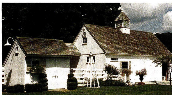
Country Carpenters built this 28x36-ft. post-and-beam-constructed barn and adjoining 9x11-ft. garden shed.
