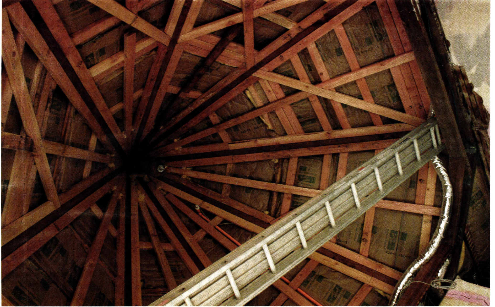
When Blahut removed the 8-ft. plaster ceiling, bracing and other framing in the Dome Room, he found a wood structure. To reinforce the vaulted ceiling, he ran a pair of steel cables through the lower perimeter of the roof's hip rafters, and then trussed the underside of each of the eight faces of the dome. Photo: Williams Cottage Inn Management
