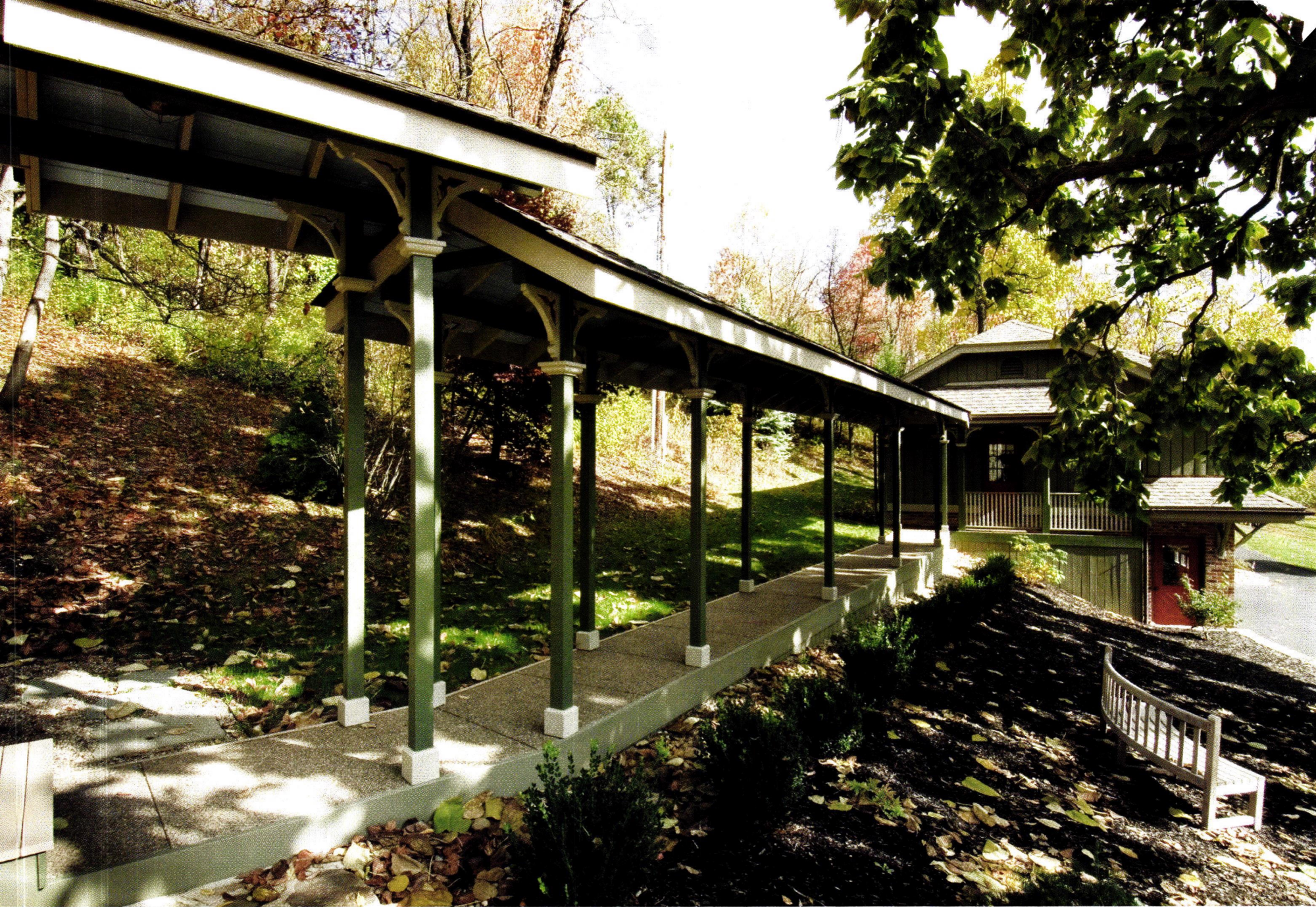
Stepping down slightly from the main house, the covered walkway extends over 60 ft. to the carriage house; its bracket details mimic those on the original porch of the main house. Photo: Craig Thompson
