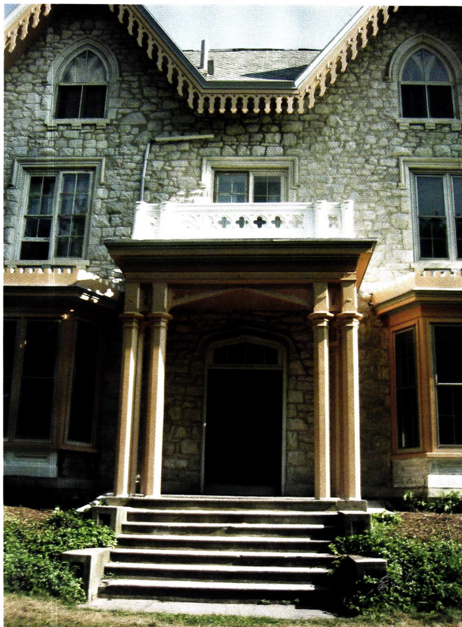
Above: Trios of faceted columns support a rebuilt section of Lovat's verandah with a quatrefoil-pattern balustrade, flanked by faceted bays with restored rail-and-stile panels (long hidden under plywood) and castellated crowns.
