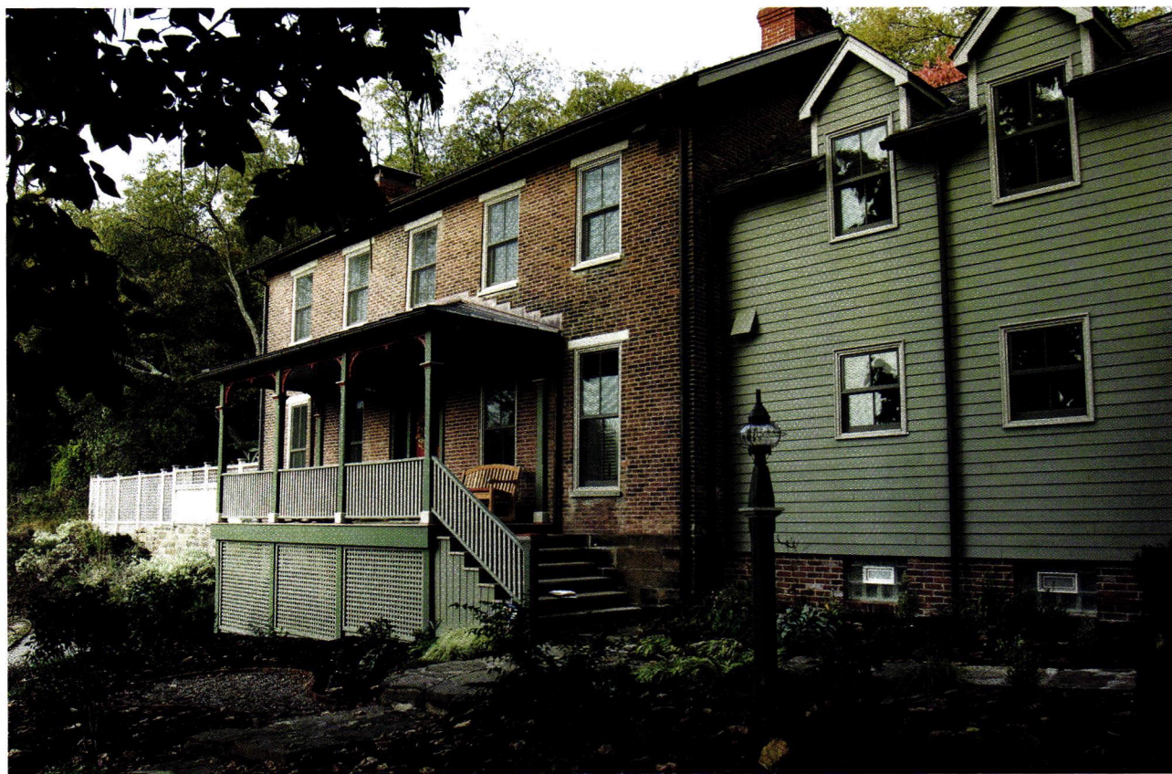
The main house, constructed in the 1840s, has a symmetrical five-bay-wide, center-hall plan typical of farmhouses of the region. The wood addition, which was built in the 1970s, is now finished with HardiPlank clapboard siding and topped with CertainTeed shingles. Photo: courtesy of Cochran Associates Architects
