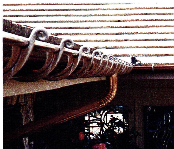
This decorative 6-in. half-round gutter from Classic Gutter Systems is made of 20-oz. copper and heavy-duty aluminum.
