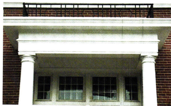
Molded fiberglass elements from Architectural Fiberglass Corp. were used to replicate historical moldings for this residence.
