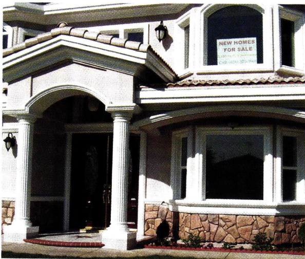
A&M Victorian Decorations' foam molding was used for the arched entry trim, window trim, sills and cornice moldings on this house.
