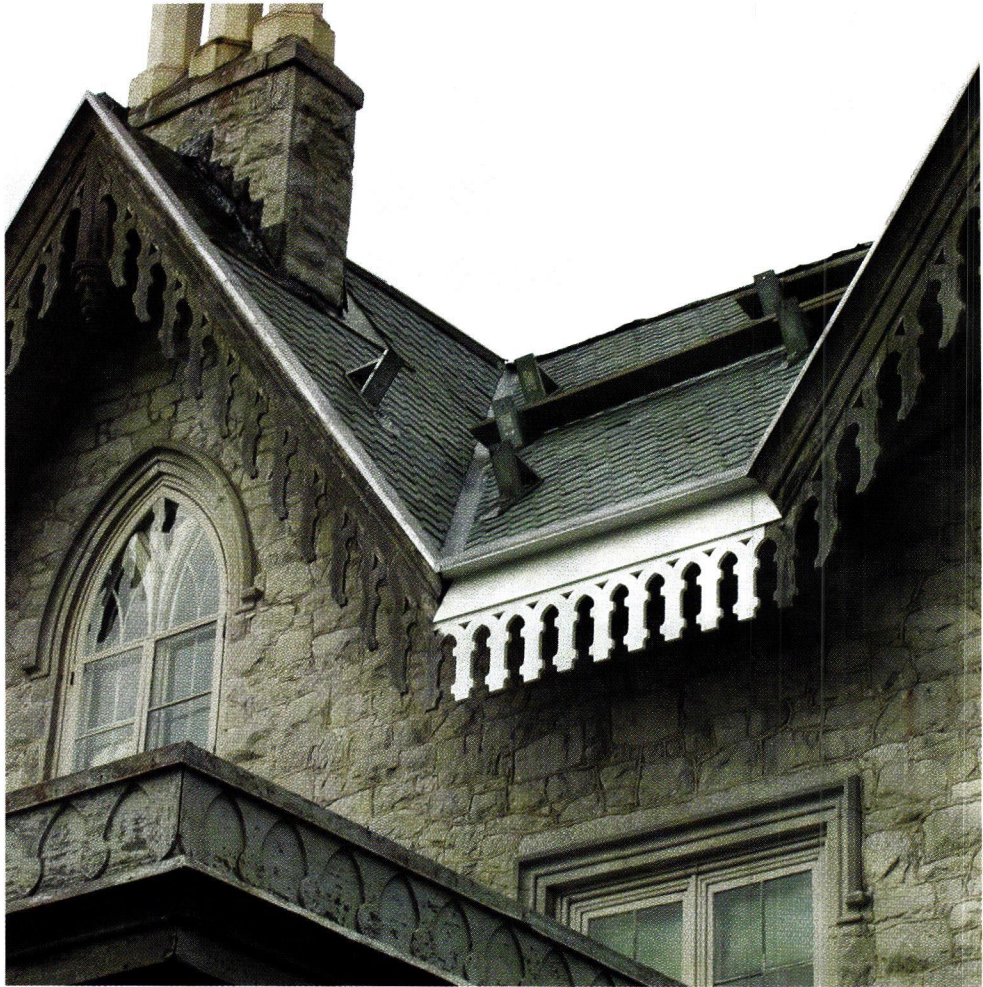
Above: About 20 percent of the marble walls required repointing, with soft lime mortars of types N and O that resemble 1850s formulas. Right: Partway through the multi-phase construction project, new cedar bargeboards contrasted with their weathered ancestors.
