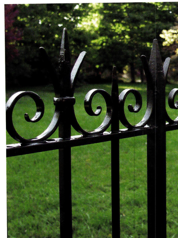
This custom fence was designed and fabricated by Wiemann Ironworks using solid-bar steel; to ensure longevity, it was galvanized before urethane coating was applied.
