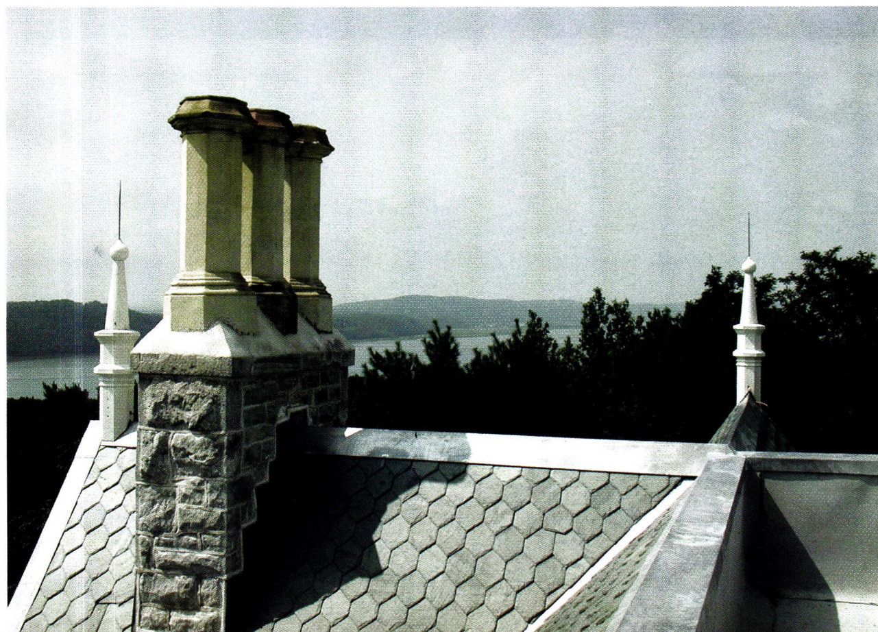
Lovat's complicated roofline, with spectacular Hudson River views, sports new wooden finials, slate hexagons and lead-coated-copper flashing, alongside 1850s terra-cotta chimneypots.
