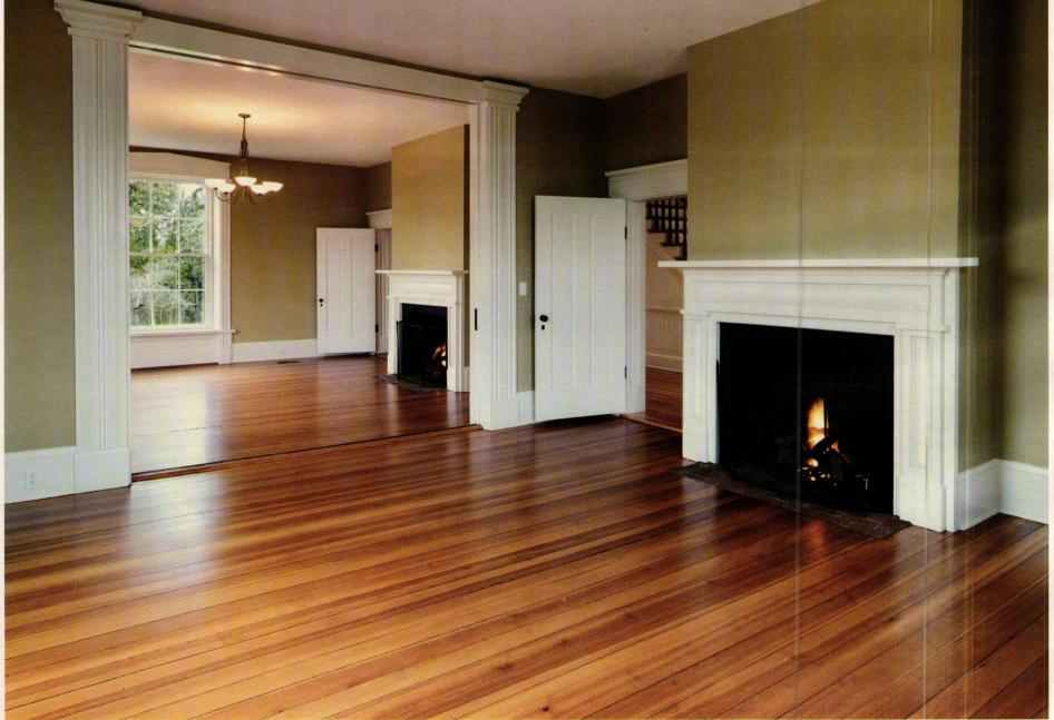
The bad bricks on all the fireplaces were replaced using lime-based mortar. Antique heart-pine floors were refinished throughout.
