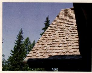
Fire-treated western red cedar roof shakes from Bear Creek Lumber were installed on this roof.
