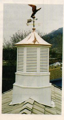
This 4x7-ft. cupola with PVC-coated aluminum cladding was restored onsite by New Concept Louvers.
