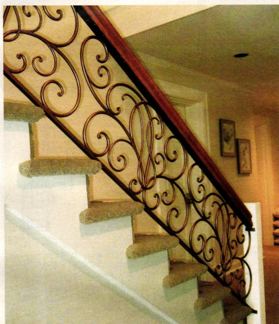
The scroll lines of this staircase by Fine Architectural Metalsmiths were forged with tapered fern-frond scroll endings and finished with a copper patina.
