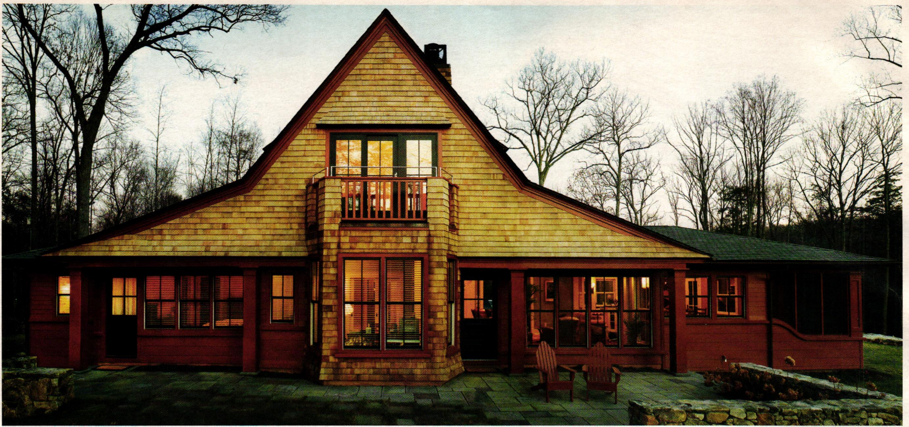
Above: The first floor of this DPA-designed house in Carmel, NY, is finished in wood trim, while the second floor and distinctive winged gable are shingled.
