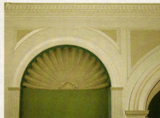
Cornice #6310 and niche cap #7821 from Felber Ornamental Plastering Corp. were used in this custom wall installation.
