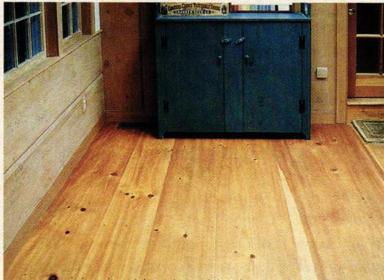
Wide-plank flooring from Craftsman Lumber is dried and machined on the premises.
