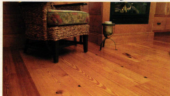
This flooring was installed using reclaimed antique heart pine in a flatsawn select grade supplied by Longleaf Lumber.
