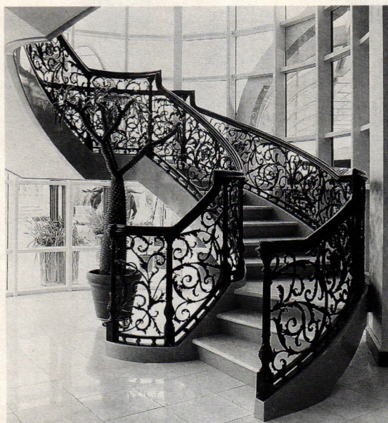
This bronze staircase was custom fabricated by Historical Arts & Casting for a residence in Sacramento, CA.
