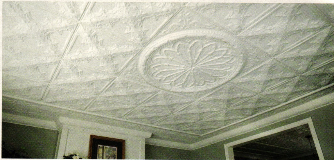
The raised, embossed decoration of many tin ceiling patterns makes the perfect canvas for faux-painting, too, Brian Greer's Tin Ceilings, Walls & Unique Metal Work
