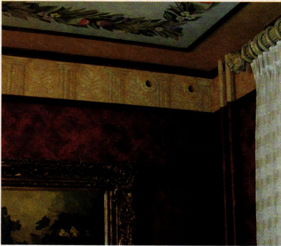
Unico's small-duct, high-velocity HVAC system takes less than 1/4 the space of a traditional system, making it ideal for historic buildings.
