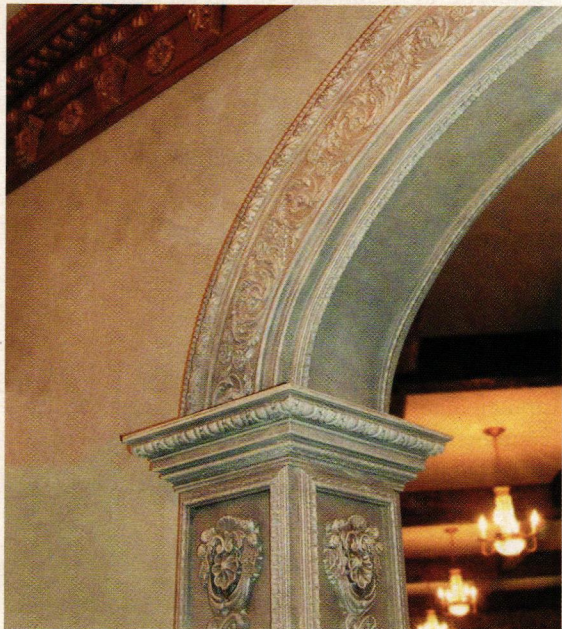
Goodwin Associates supplied this faux-finish entryway with decorative gold-leaf molding.
