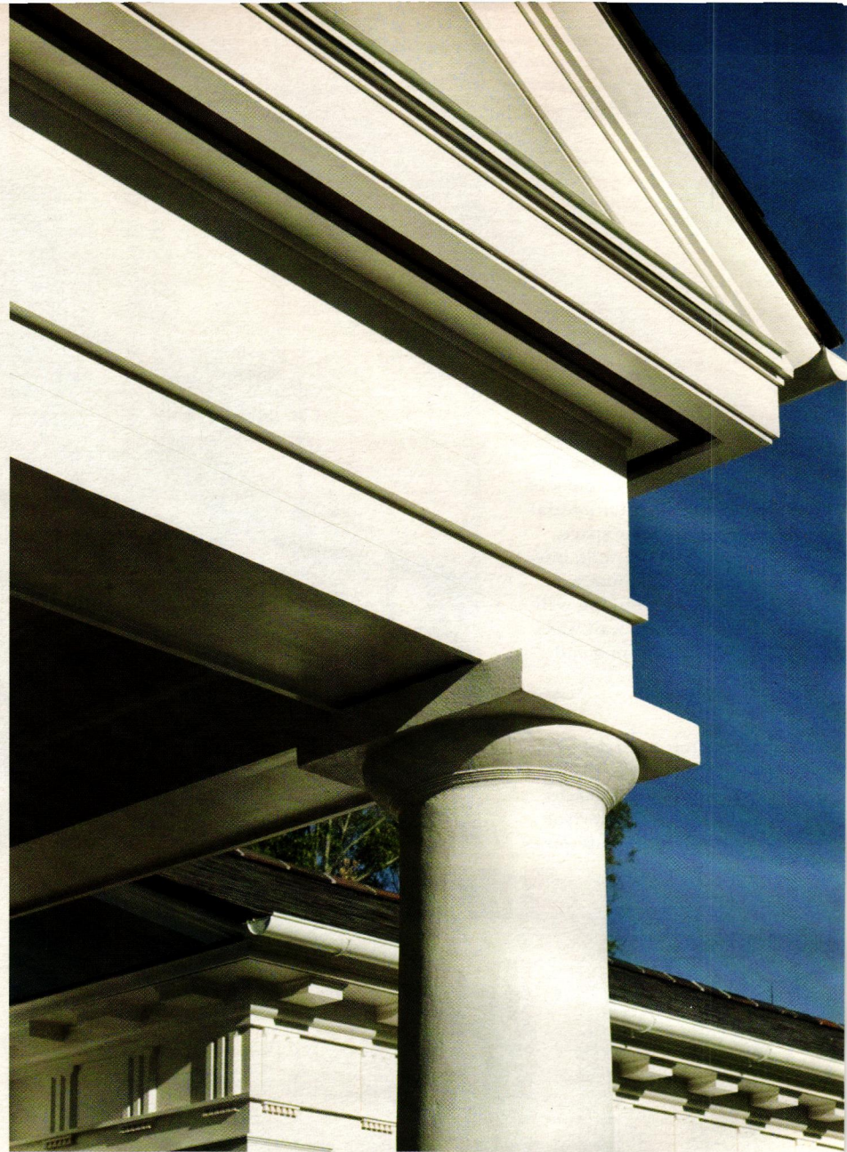
Above and above left: The pool house pediment is supported by masculine Greek Doric columns, which were constructed using traditional methods: stacked bricks with a stucco overlay. The bricks used for the terrace are queen-sized Carolina handmade brick.
