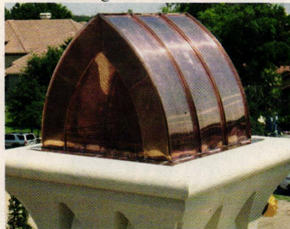
EJMcopper fabricated this chimney cap, which includes a bug screen.
