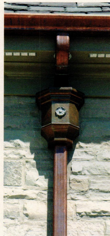
The traditionally styled Royal conductor, available from RainTrade, is made of 16-oz. copper with a cast-brass rosette; it is available in two sizes.
