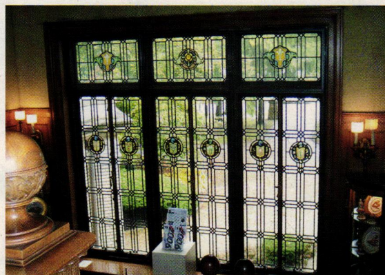
An interior storm from Climate Seal provides insulation while protecting the appearance of this historic window.
