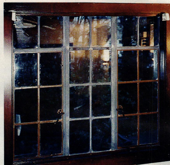
Seekircher, a specialist in steel casement-window adjustment and restoration, rebuilt this window after it was damaged in a storm.
