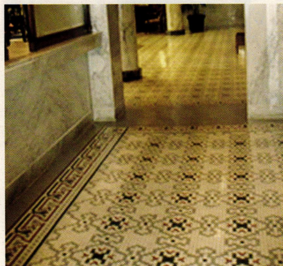
American Restoration Tile manufactured this 1-in. hexagonal, unglazed porcelain flooring tile.
