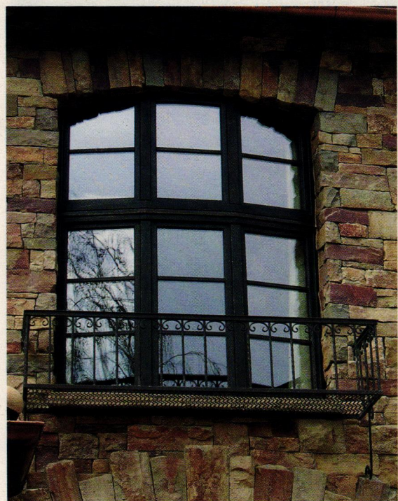
This custom bronze-clad tilt-and-turn window was fabricated by Grabill; it has an antiqued patina and an aged-wood interior.
