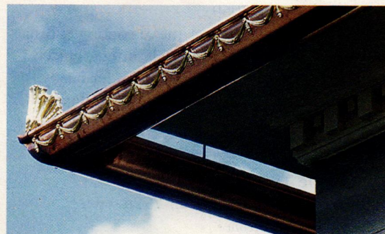
Classic Gutter Systems fashioned this elaborate half-round copper gutter with gold-patinated solid-brass trim and a rain deflector.
