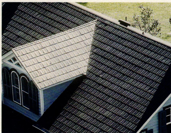
Conklin Metal Industries offers metal shingles in its 10x14-in. Diamond Stamped Pattern in six types of metal.
