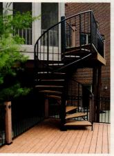
Goddard's custom spiral stairs are available in wood, steel or a combination of both; steel stairs are of welded one-piece construction.
