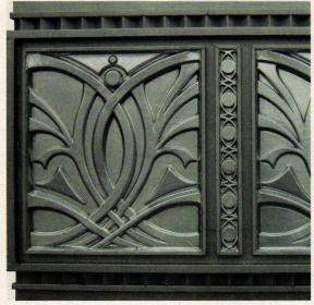
NIKO fabricated this custom zinc spandrel panel for a building in Washington, DC.
