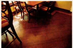
Made of cork supplied by Globus Cork, this floor is designed to look like traditional wood flooring.
