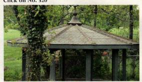
This gazebo features W.F. Norman Corp.'s Style "A" shingles with its continuous hip finish and a custom-made finial on top.
