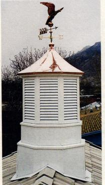
This 4x7-ft. cupola with PVCcoated aluminum cladding was restored onsite by New Concept Louvers.
