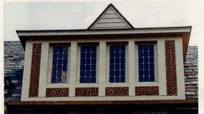
These 75-year-old steel casement windows were salvaged and then incorporated into this structure by Seekircher Steel Window Repair.
