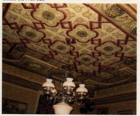
This Oriental-style ceiling was created using pressed-tin panels from W.F. Norman Corp.
