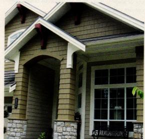
Nichiha's ½-in.-thick fiber-cement shakes create shadow lines similar to traditional wood siding.
