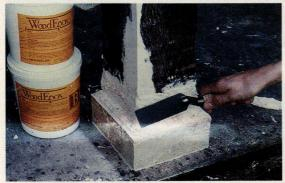
WoodEpox from Abatron can be used to repair wood elements such as this column.
