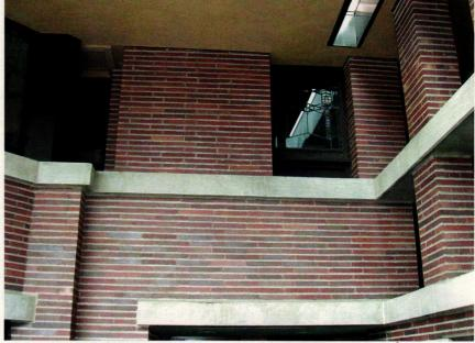
Wright's clever use of mortar to emphasize horizontality becomes clear on the newly re-pointed East elevation, where the natural-color bed joints stand out but the red vertical joints blend in with the bricks.
