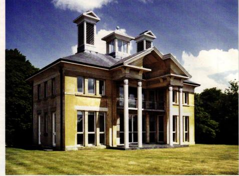
The south elevation of Robert Adam's solar house features large areas of triple glazing for solar gain. The attenuated columns, which minimize interference with solar rays, were inspired by fantasy architecture in Pompeian wall paintings. The pediment breaks back dramatically in the center to admit low winter sun that heats the thermal mass inside, including the black slate floor.
