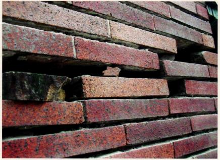
A detail of the chimney gives a clear view of the tile-like Roman brick so favored by Wright, as well as typical masonry damage due to water intrusion.
