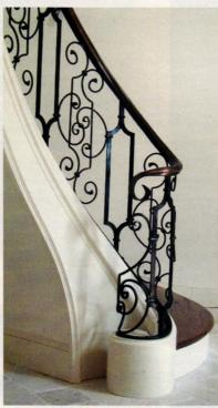
This railing with artful scrollwork was custom fabricated by Schwartz's Forge & Metalworks.
