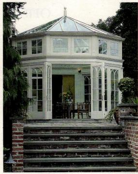
Built by Tanglewood Conservatories, this glass house features woodwork on the interior and maintenance-free aluminum cladding on the exterior
