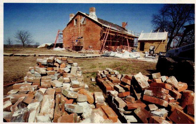
More than 10,000 handmade bricks were salvaged from a neighboring house, which dated from 1842 and had been demolished in the '70s. The brick allowed the team to re-create the original window openings, which had been altered in the mid-20th century. Photo: Rob Hill
