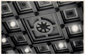
NIKO fabricated and installed these pressed-metal coffers.
