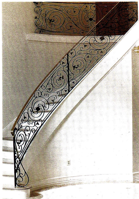
This railing from Fine Architectural Metalsmiths features French Country-style scrollwork with bronze leaf finials and center rosettes.
