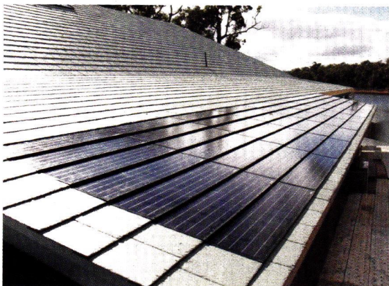
Greenstone Slate offers energy-saving roofing such as this natural Vermont slate installation with integrated solar panels.
