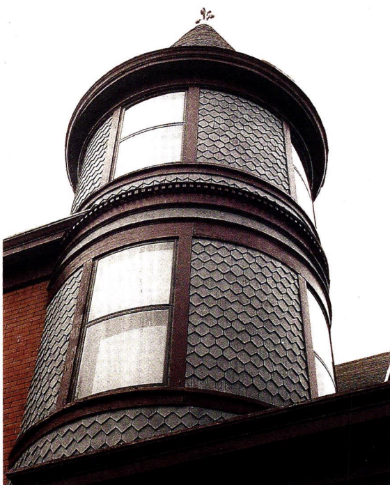
Allied Window designed and fabricated the bowed storm windows for this historic home.
