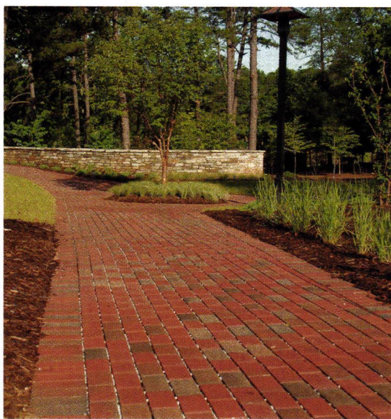
Pine Hall Brick's StormPave permeable clay paver allows rainwater to filter down through a specially constructed paving system and dissipate into the soil, rather than carry excess pollutants into storm drains; it contains 53% pre-consumer recycled content.
