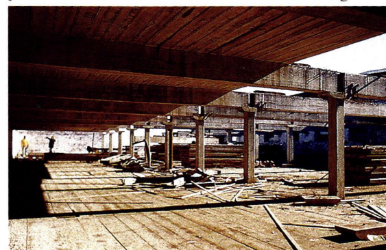
Longleaf Lumber salvaged and recycled the old-growth timber from this building.
