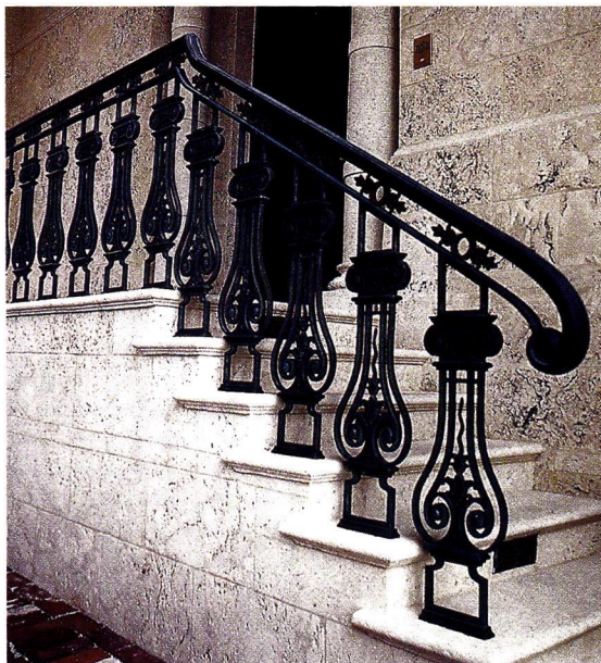
Historical Arts & Casting fabricated this traditionally styled, cast-bronze railing.
