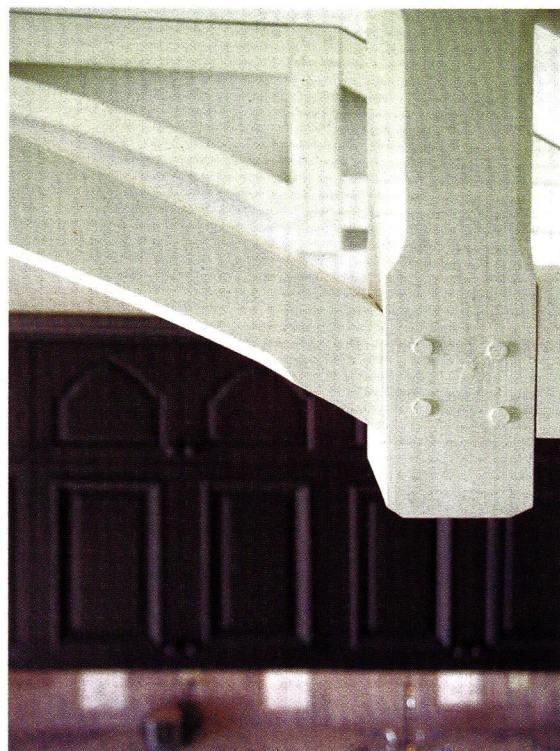
This brace detail from a structural truss shows the work of Hugh Lofting Timber Framing.
