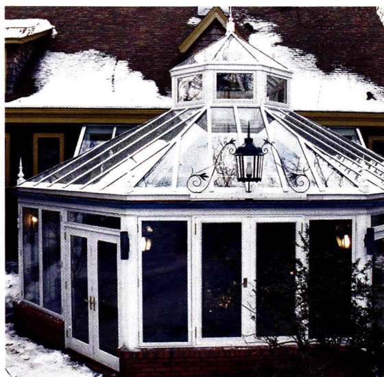
This lantern-roof conservatory by Glass House has an aluminum-clad exterior, which provides a weatherproof barrier for the wood frame.
