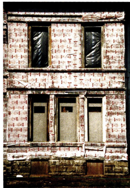
Dumond Chemicals' Peel Away paste and Peel Away cloth were applied to this masonry building to remove the existing paint.
