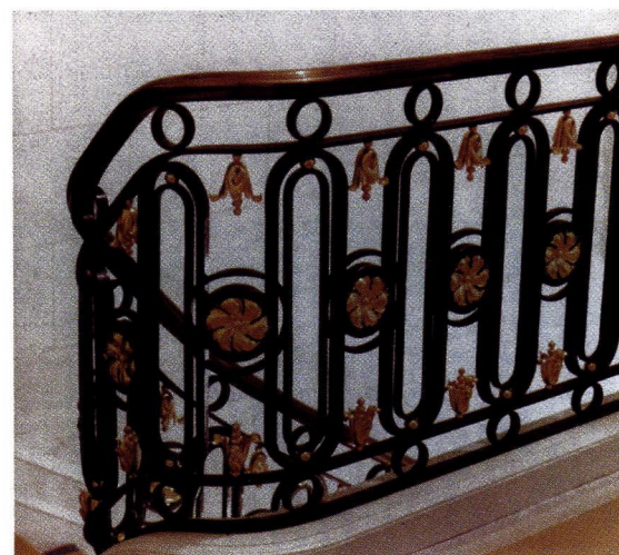
This stair balustrade, fabricated by Schwartz's Forge & Metalworks, has gilded repousse leaf work and a custom bronze cap rail.
