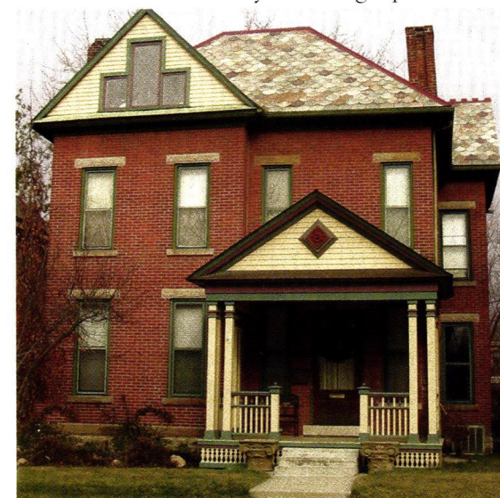
Durable Slate installed this slate roof using reclaimed Vermont semi-weathered gray-green and purple slates.
