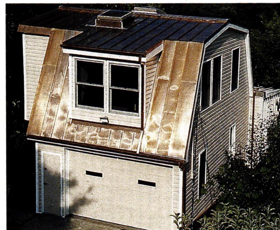
NIKO Contracting installed the copper standing-seam roof on this carriage house.
