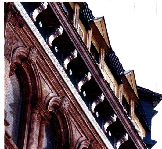
This stamped sheet-metal cornice was fabricated by W.F. Norman.
