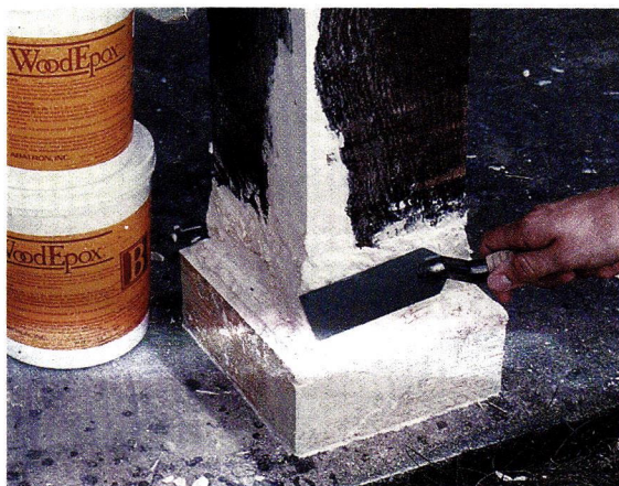
WoodEpoxy from Abatron can be used to repair wood elements.
