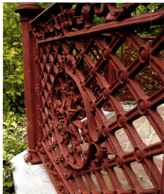
This detail is from a cast-iron gazebo that was recast and fabricated by Wiemann Metalcraft.
