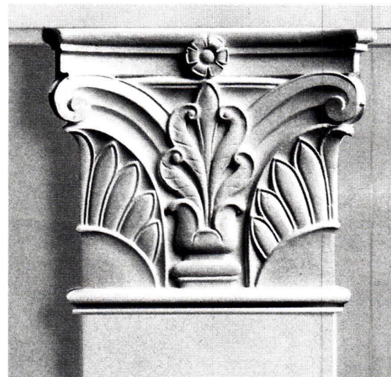
This plaster capital from Felber Ornamental Plastering Corp. measures 6½ in. tall x 6¾ in. wide and projects ⅝ in.
