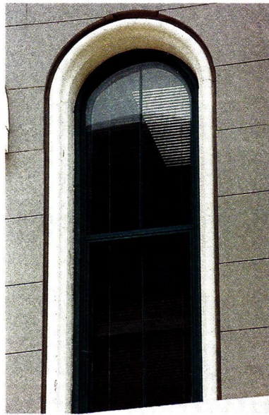
Allied Window's HOL-B Historic-One-Lite exterior storm windows were installed on the 4th and Plum apartment building in Cincinnati, OH.
