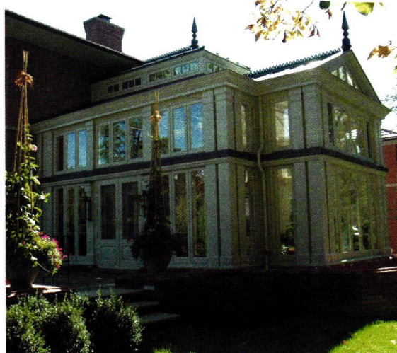
This dramatic two-story conservatory with a soaring lantern roof is anchored by double corner columns; it was custom designed and fabricated by Oak Leaf Conservatories.
