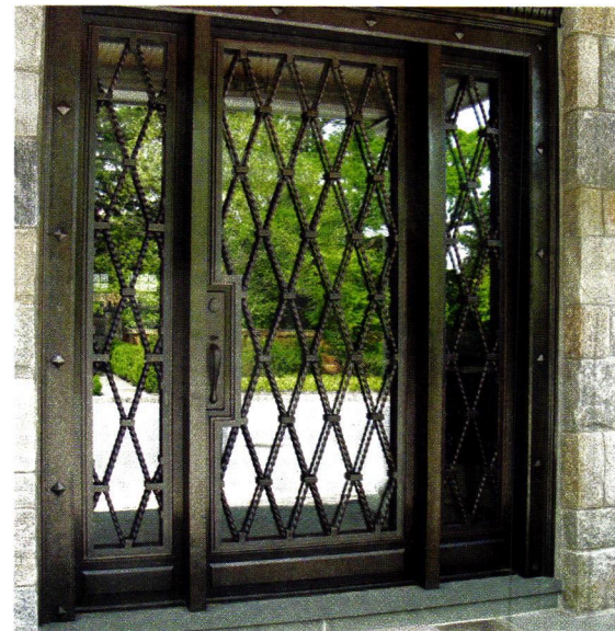
Wiemann Metalcraft fabricated this bronze door with insulated glass.
