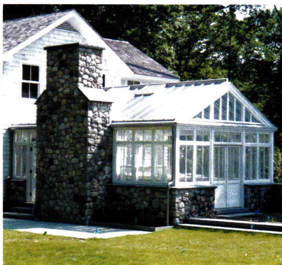
This Classic conservatory designed by Glass House, LLC, features mahogany framing, true-divided-lite windows and doors, automated ridge vents and a shading system.
