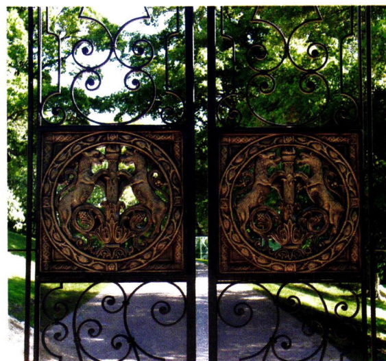
A landmark masonry element was re-cast and bronzed by Fine Architectural Metalsmiths to create these dramatic medallions for a monumental driveway gate.
