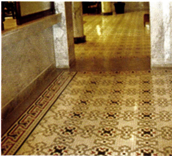
American Restoration Tile manufactured this 1-in. hexagonal, unglazed porcelain flooring tile.
