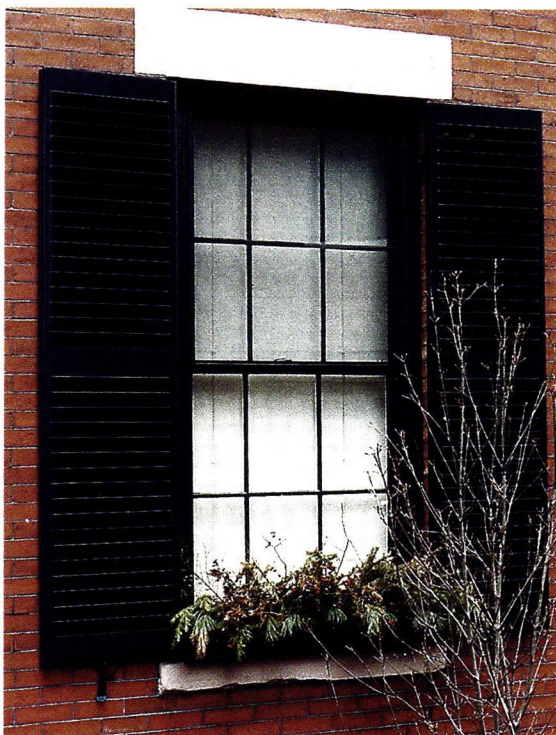
Beech River Mill manufactured these 1 3/4-in.-thick shutters that feature a 2 3/4-in.-wide fixed slat with scalloped corners projecting beyond the face of the frame stock.
