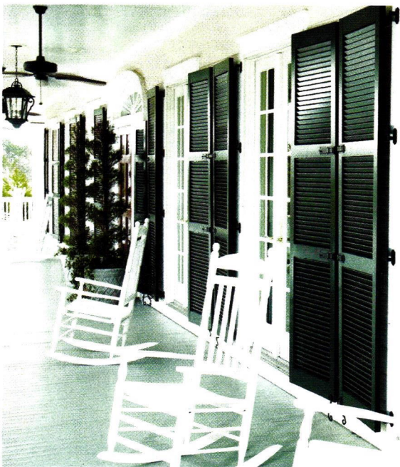
Historically accurate shutters from Atlantic Premium Shutters are made of high-density PVC and composite wood to resist harsh weather.
