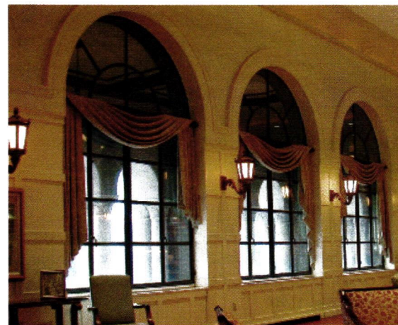
Steel Windows & Doors supplied these W20 series hot-rolled steel windows by Crittall Windows.
