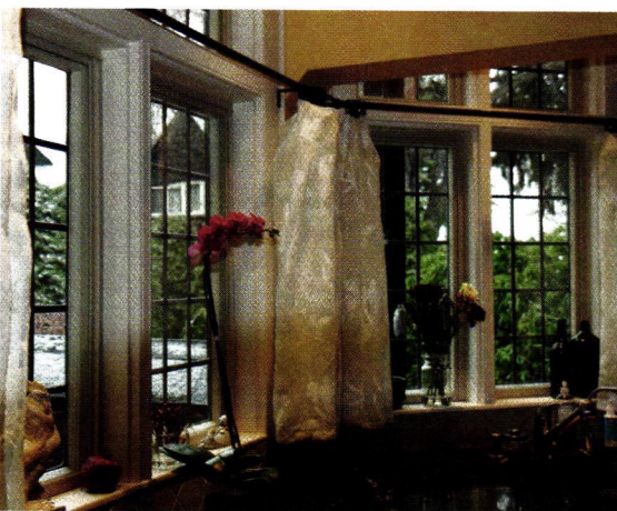
These historic windows now have interior glass storm windows from Innerglass Window Systems.
