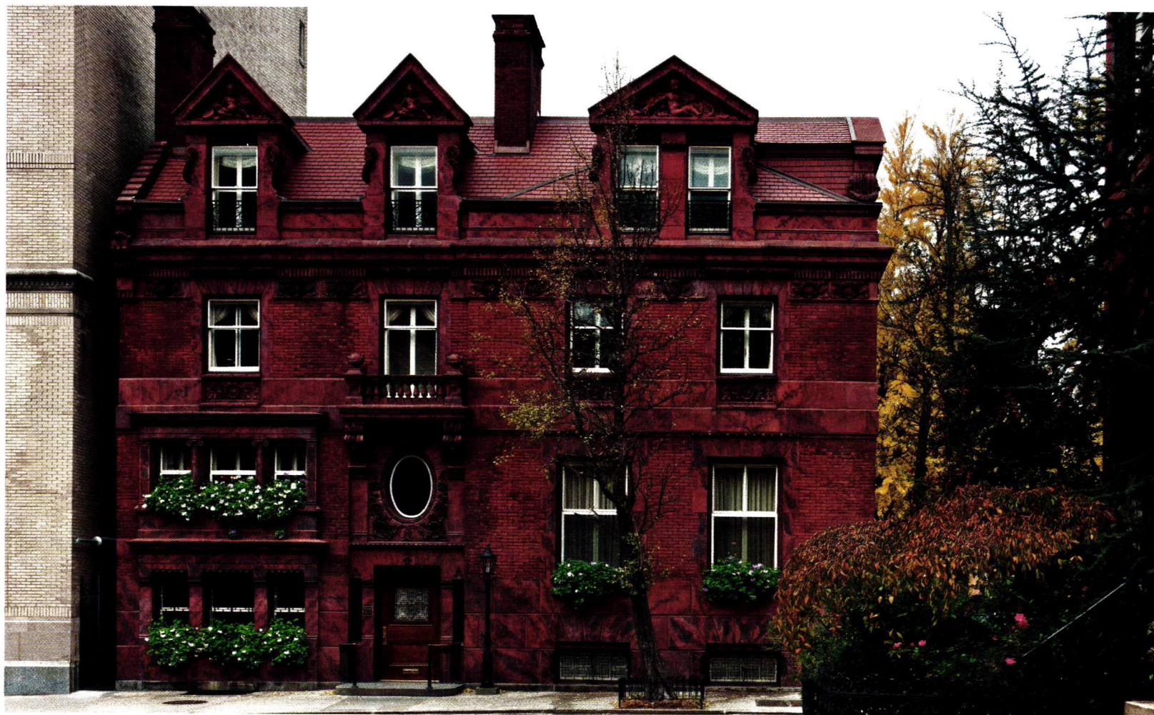
New terra-cotta roofing tile tops the restored masonry façade, with its brick and sculptural terra-cotta elements. The comprehensive exterior transformation also included the restoration of original windows and the flagstone stoop. All Photos: Tom Crane Photography
