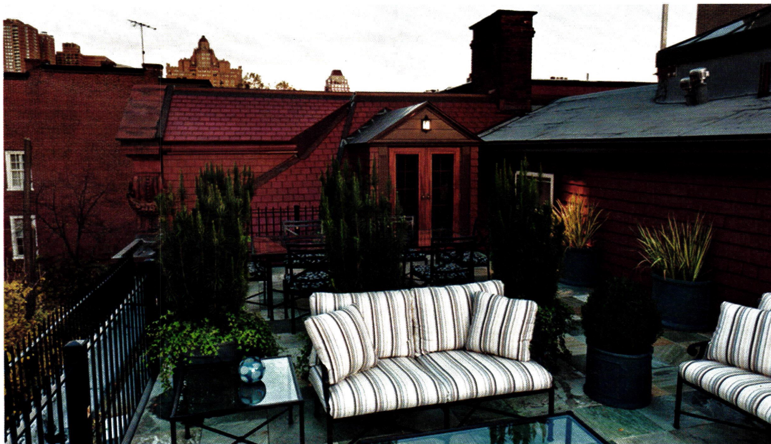
After a 1980s roof deck was removed, a new membrane roof was installed and topped with a flagstone terrace on a pedestal paving system.
