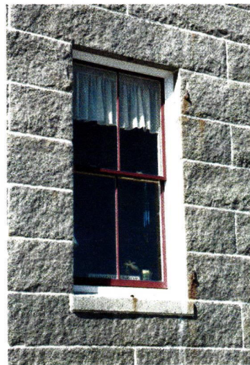
Architectural Components restored the double-hung windows to match the brick molding detail for the Customs House Maritime Museum in Newburyport, MA.
