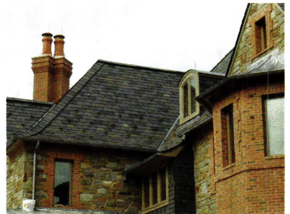
Reclaimed Roofs supplied a blend of new Vermont Gray and Gray-Black slate for this roof in Chadds Ford, PA.
