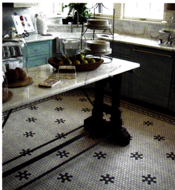
This historically accurate floor was created using 1-in. hexagon unglazed porcelain tile and 3/4-in. square border tile from American Restoration Tile.
