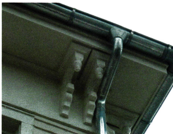
Ornametals supplied the standing-seam gray zinc roofing and rainwater system for the historic antebellum Cooper House in Huntsville, AL.
