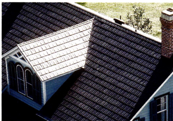
Conklin Metal Industries offers shingles in its 10x14-in. Diamond Stamped Pattern in six types of metal.
