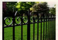
This custom fence was designed and fabricated by Wiemann Metalcraft using solid-bar steel; to ensure longevity, it was galvanized before urethane coating was applied.
