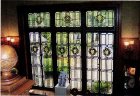
An interior storm from Climate Seal provides insulation while protecting the appearance of this historic window.
