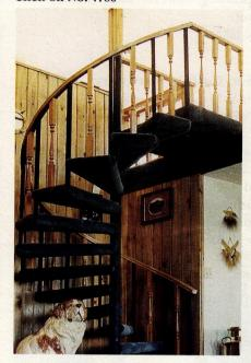
Fabricated by Goddard Spiral Stairs, this metal and wood staircase features center balusters of oak and solid-wood handrails.
