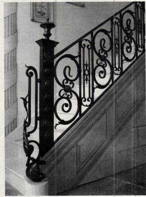
This custom-forged, cast-bronze and -iron stair railing was fabricated by Wiemann Metalcraft.
