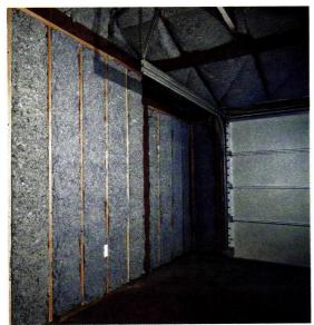
UltraTouch Denim Insulation is made of recycled cotton by Bonded Logic of Chandler, AZ.
