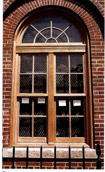
This double-hung window unit with a fixed-arch fan was constructed by  $\mbox{\bf Artistic}$ Doors & Windows with mortise-andtenon joinery. .
