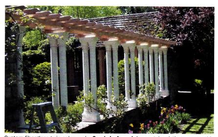
Custom fiberglass twin columns by  ${\bf Goodwin\ Associates\ }$  match existing ones on this restored pergola.
