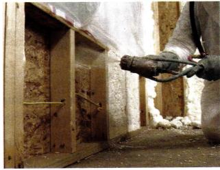
Spray polyurethane foam from BioBased of San Diego, CA, integrates soy as a replacement for a portion of the petroleum traditionally used in the product.
