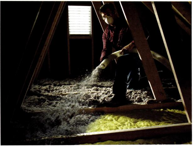
This loose-fill cellulose insulation is made from recycled newspapers by Charlotte, NC-based GreenFiber.
