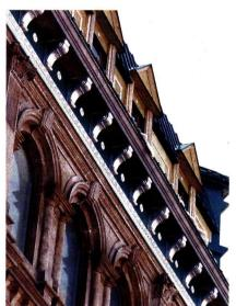
This stamped sheet-metal cornice was fabricated by **W.F. Norman**.
