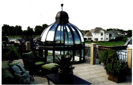
This dome skylight from **Solar Innovations** utilizes 1-in. insulted glass and solid copper and bronze panels.
