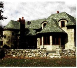
This graduated Vermont roofing slate from Greenville, DE-based Reclaimed Roofs was salvaged from a university building and re-installed on this residence in Connecticut.
