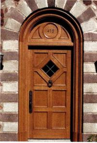
**HeartWood Fine Windows & Doors** fabricated this 21/4-in. thick mortiseand-tenon solid-wood door out of sawn white oak to replicate the original door made 100 years ago.
