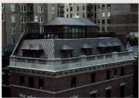
NIKO fabricated the copper dormers and mansard roof and also installed the copper penthouse for this building in New York City.
