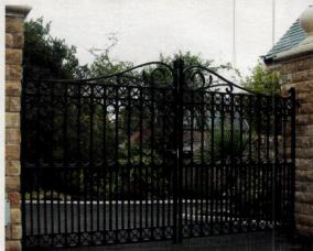
This iron gate for a 12-ft. opening was cast in one piece by Wiemann Metalcraft; it was installed on in-ground hydraulic operators.
