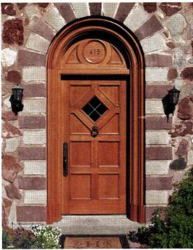
HeartWood Fine Windows & Doors fabricated this 2½-in. thick mortise-and-tenon solid-wood door out of sawn white oak to replicate the original door made 100 years ago.
