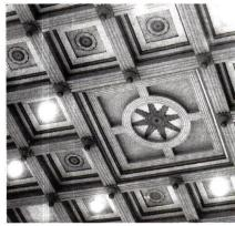
NIKO fabricated and installed these pressed-metal coffers.
