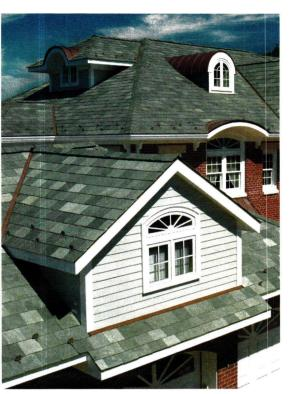
TruSlate roofing from GAF combines traditional slate with a hightech waterproofing material.
