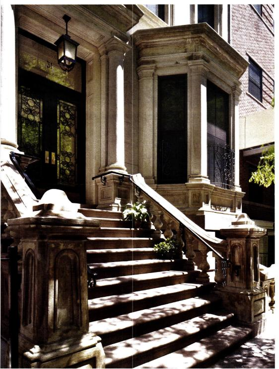
The exterior was cleaned using micro-abrasion and chemical peeling, and excess cement was removed to reveal the articulation of the stone column capitals and pediments.
