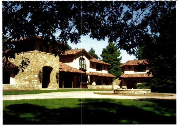
Tile Roofs supplied the salvaged-clay Mission-style tile for the roof of this home in the Kansas City area. Photo: courtesy of Tile Roofs
