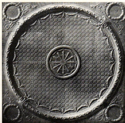
Empire Center, model #8706 from W.F. Norman, is composed of eight ceiling plates, each measuring 24x48 in.
