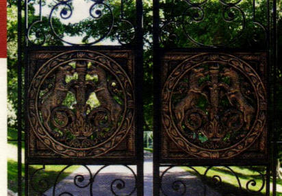
A landmark masonry element was re-cast and bronzed by Fine Architectural Metalsmiths to create these dramatic medallions for a monumental driveway gate.
