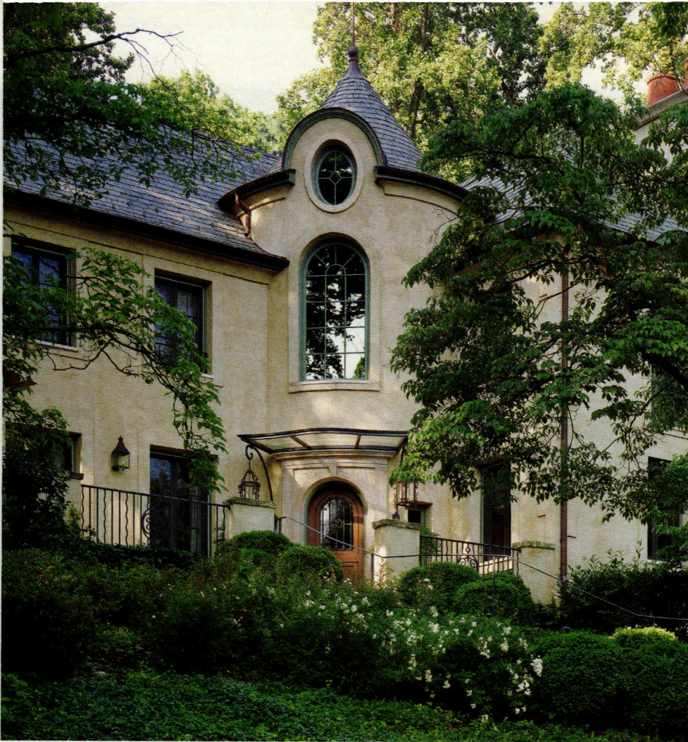
ABOVE: A renovation by Barnes Vanze Architects tripled the size of a residence in Washington, DC's Foxhall neighborhood. The original house, ca. 1920, was gutted, and a two-story wing was added. Its original brick tower was covered with stucco.
