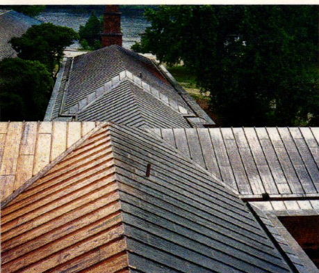
NIKO Contracting Co., Inc. installed this batten-seam and flat-lock copper roof.
