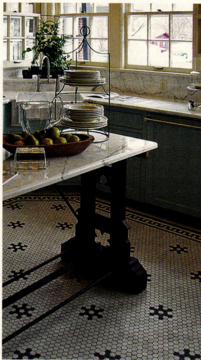
This historically accurate floor was created using 1-in. hexagon unglazed porcelain tile and 3/4-in. square border tile from American Restoration Tile.
