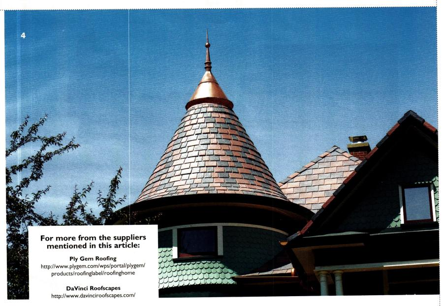
1. Ply Gem Roofing manufactures its engineered slate using a process called Fusion Annealing (applying low heat and high pressure).
