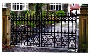
This iron driveway gate for a 12-ft. opening was cast in one piece by Wiemann Metalcraft; it was installed on in-ground hydraulic operators.
