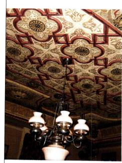
This Oriental-style ceiling was created using pressed-tin panels from W.F. Norman Corp.
