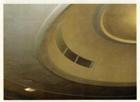
**Artistry in Architectural Grilles** manufactures the plaster "J-Bead" framed linear bar; it provides a flushed, borderless installation for plaster or drywall applications. **Call for more information.**
