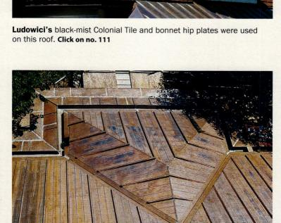
NIKO installed this batten-seam and flat-lock copper roof for an historic building. Click on no. 8300
