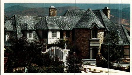
**Auburn Tile** manufactured the concrete roof tile for this custom home; it is lightweight, class A fire rated and is availabble with a slate or shake appearance in a variety of colors. **Click on no. 1518**
