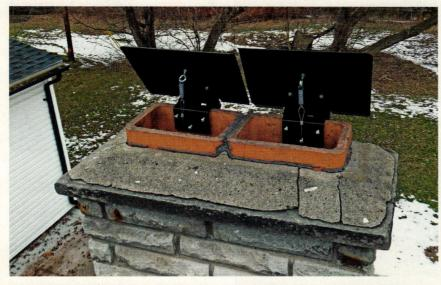
**Benson Energy's** All Season Control Cover for chimney flues can be installed with dual controls down to the firebox, one for each cover. **Click on no. 174**
