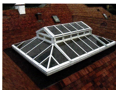
Glass House fabricated and installed this lantern hip-roof skylight with mahogany framing, aluminum cappings and flashings with motorized awning vents.
