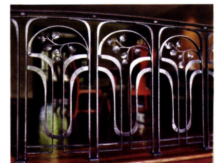
Edgar Brandt's design sensibility was the initial inspiration for this forged railing by Fine Architectural Metalsmiths ; it has an updated leaf spray and dramatic changes of dimension.
