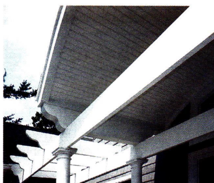
This custom pergola from Goodwin Associates uses girders and cross rafters of reinforced board that is maintenance-free and rot-resistant.
