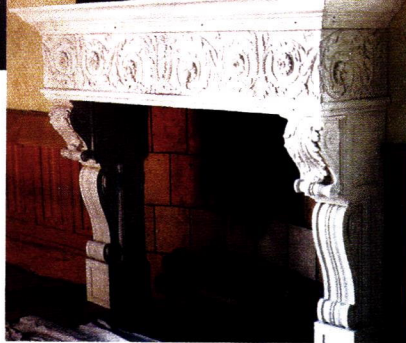
This custom Felstone mantel from Felber Ornamental Plastering Corp. was built using stock components.
