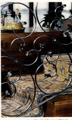
Hot-stamped leaves from **King Architectural Metals** can be used in a variety of applications; the elements adorning this railing are available in the company's catalog. Click on 270
