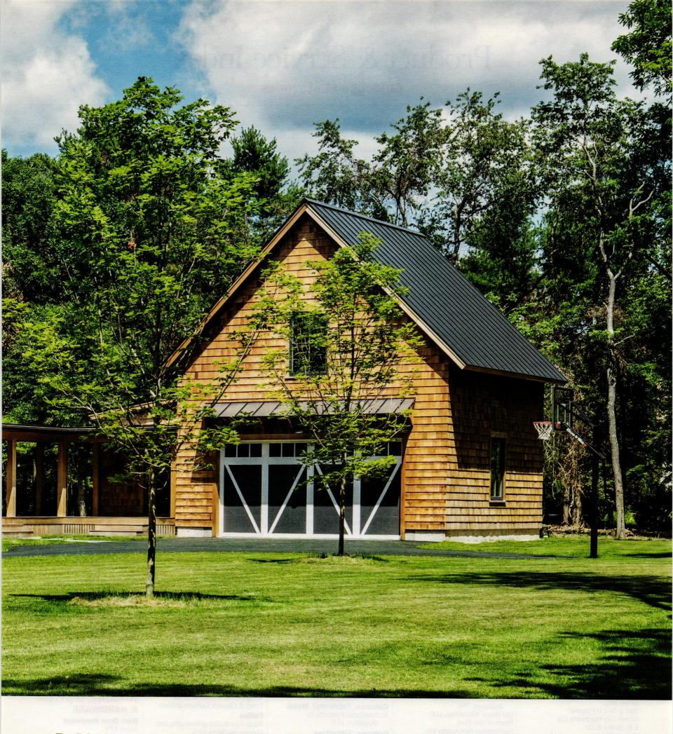
The all-electric home designed by ZeroEnergy Design consumes 70 percent less energy than a code-built house, and with measured energy data produces 48 percent more energy annually than it consumes, making it a "net positive" home. Thick walls and roofs lack thermal bridging by using dense packed cellulose and continuous rigid insulation. High performance, triple-glazed windows round out
