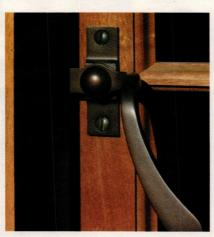
This solid-brass casement fastener from **Phelps Company** is shown in an oil-rubbed bronze finish; the firm manufactures a complete line of traditionally styled hardware for wood casement windows Click on 6001
