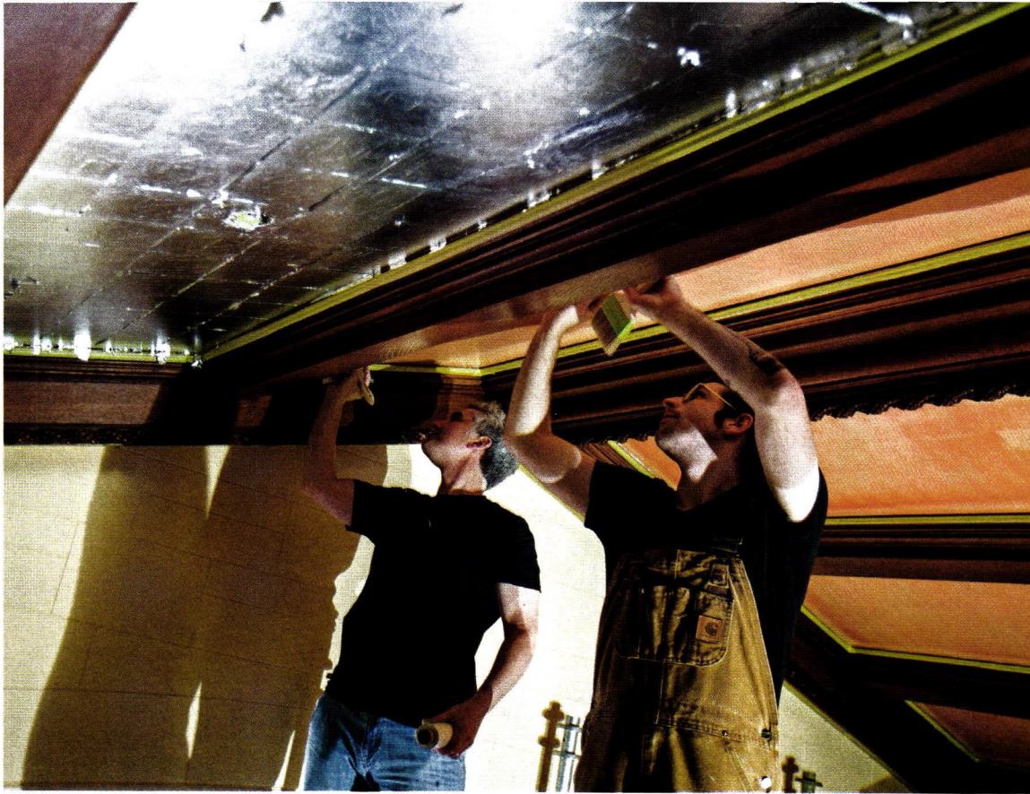
COUNTER-CLOCKWISE FROM ABOVE: Artisans from Historic Surfaces LLC apply aluminum leaf to the ceiling in Fair Lane's main hall. Photo by John F. Martin.
