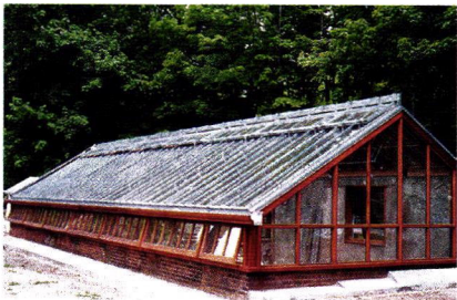
Glass House, LLC reconstructed this greenhouse that has been converted into an architectural studio; it features mahogany framing, ganged roof and side vents for ventilation, refitted with the actual chain pulley operators with copper exterior roof cappings.
