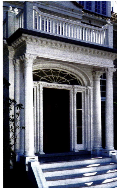
This decorative entryway showcases Chadsworth's architectural 10 in. by 8 ft. Roman Corinthian fluted wood columns and custom entablature with a walkout balcony.
