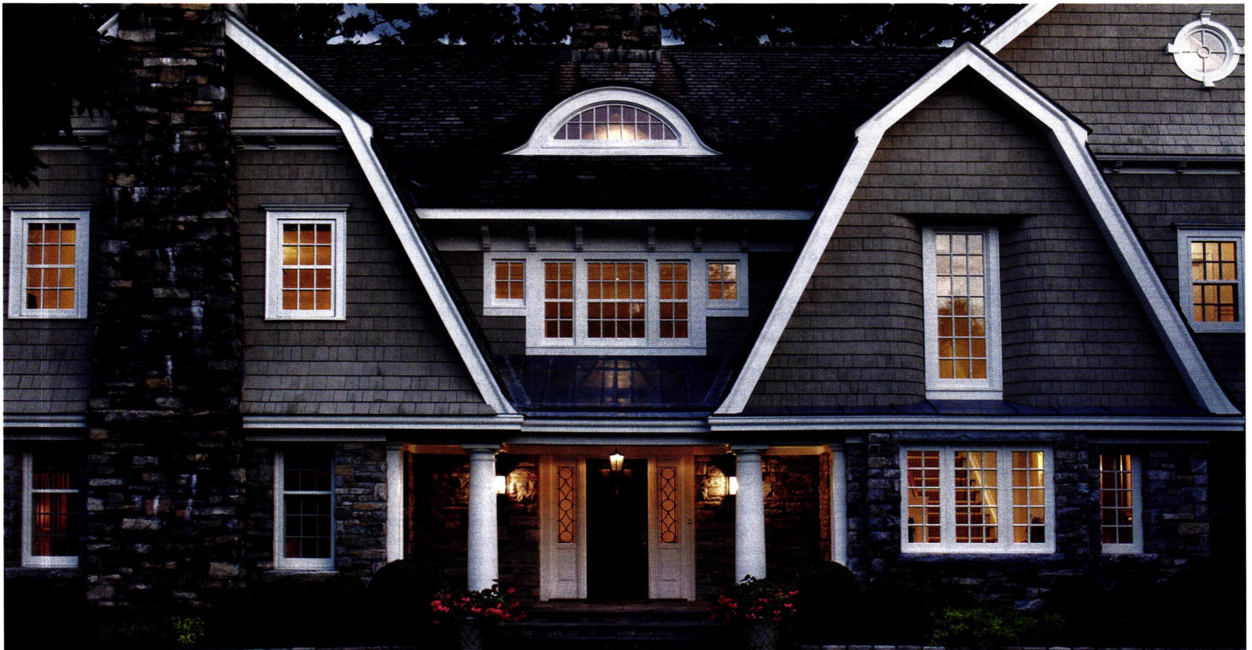
Photo courtesy of Coastal Point Development, LLC; Architect: Grandberg & Associates Architects; Photographer: Michael Biondo
