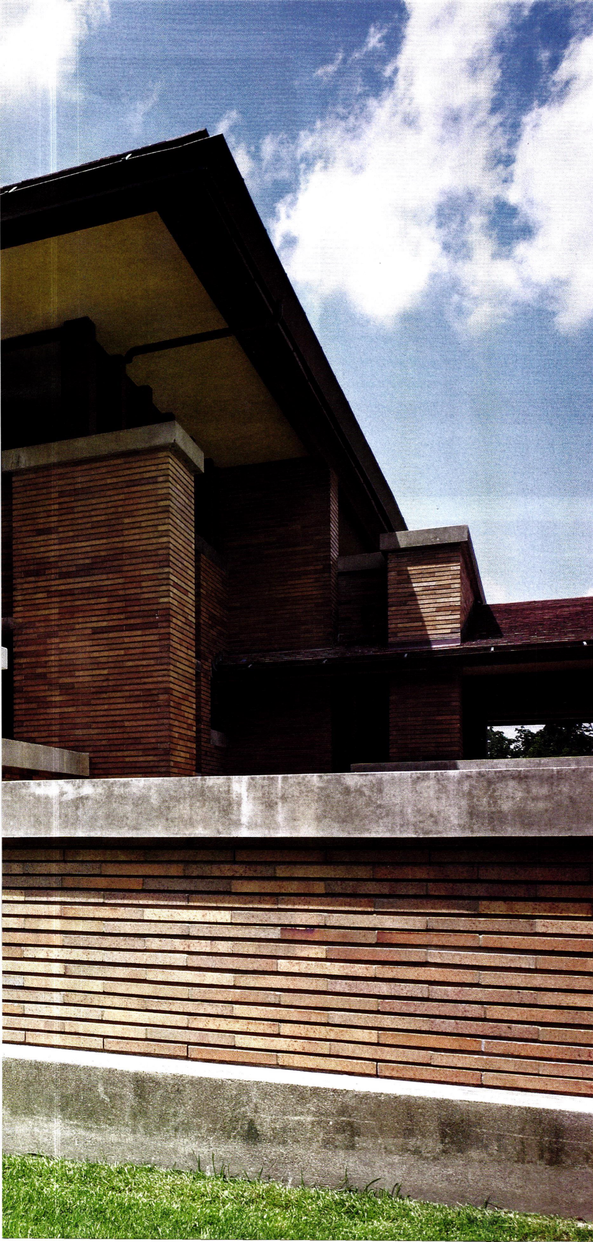
LEFT: Exterior view of Martin House with restoration complete. The new reconstructed garden wall is in foreground. Photo by Biff Henrich.
