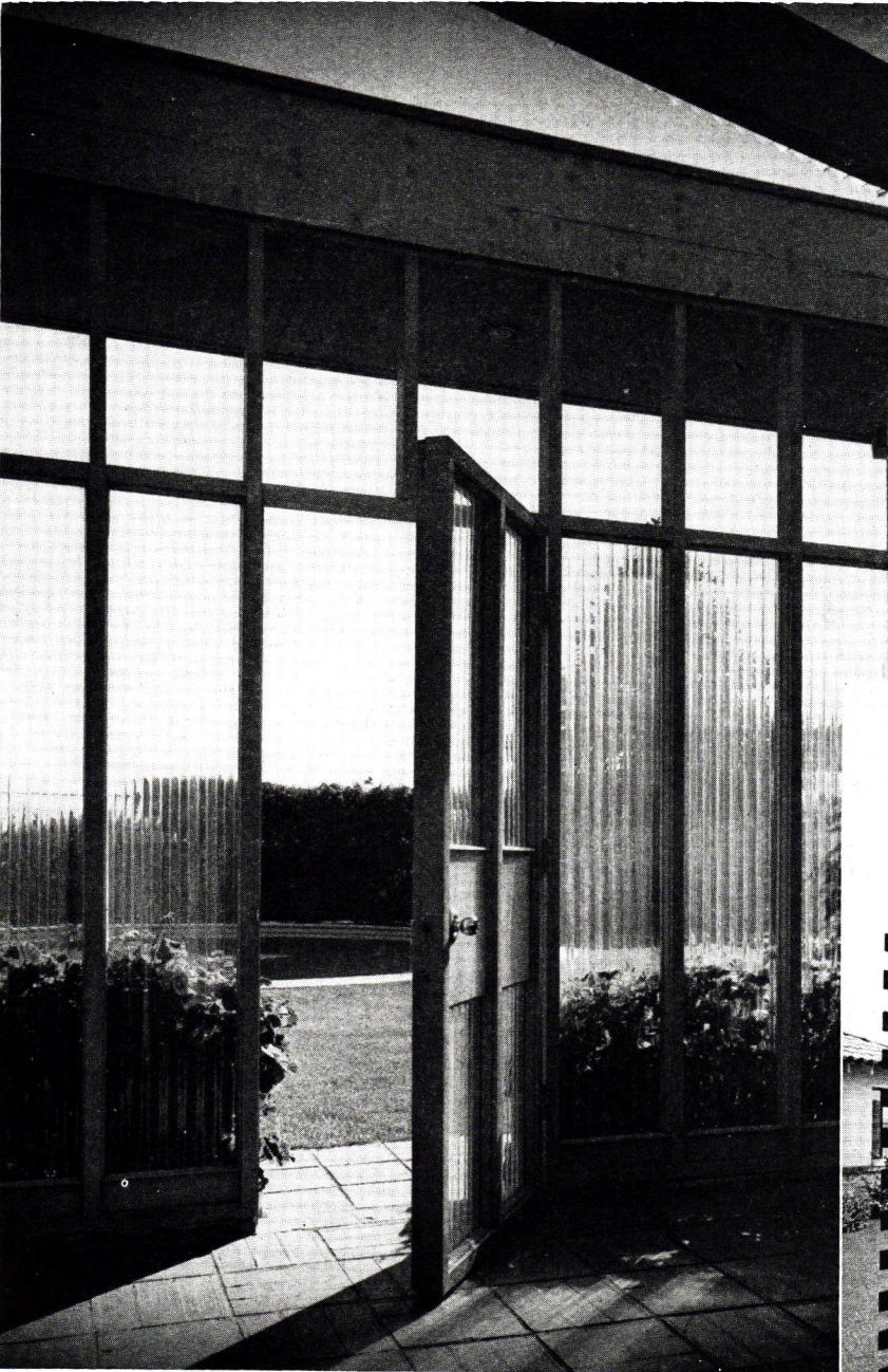
If you want a view-blocker that will not steal the light, you want structural glass or clear plastic paneling. Both are made in several patterns that diffuse and soften the light. The lower part of the wall (above) was made of corrugated panels, the top of clear glass. Hand-woven redwood strips screen entrance (right) from street
