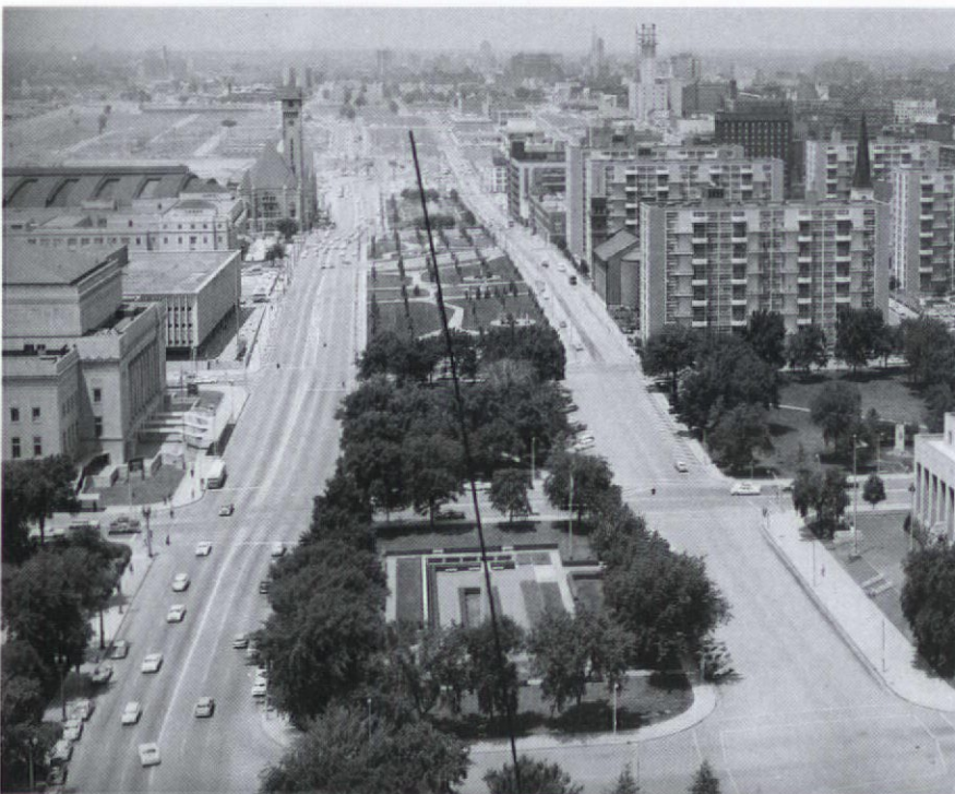
Above: The site of the Central Parkway/Gateway Mall, looking west from the site of the proposed Civic Center, before either the Parkway or Civic Center were constructed.
