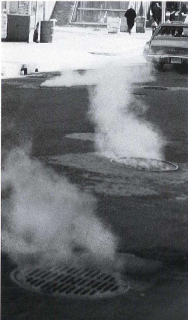
In the winter, steam clouds issue from manholes, grates and other openings.
