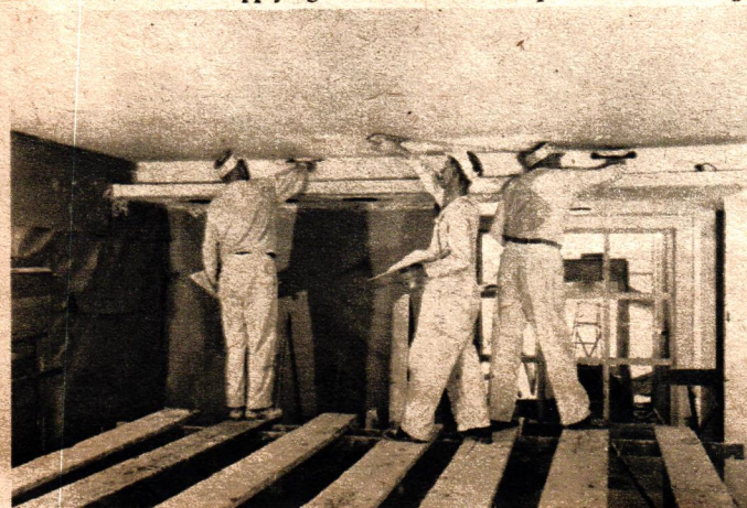
BELOW: Workmen applying SABINITE acoustical plaster to a ceiling.
