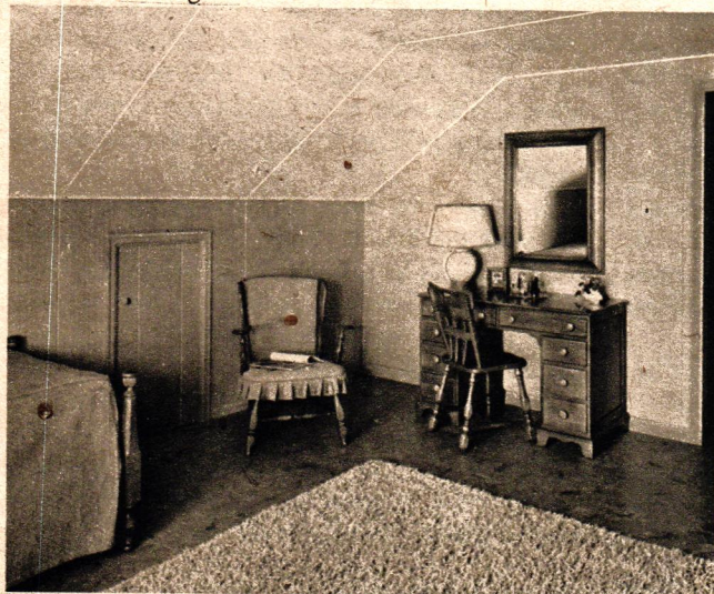
An access panel allows the lowest space below the eaves to be used for storage purposes. Built-in drawers and cabinets are another method of using this space.
